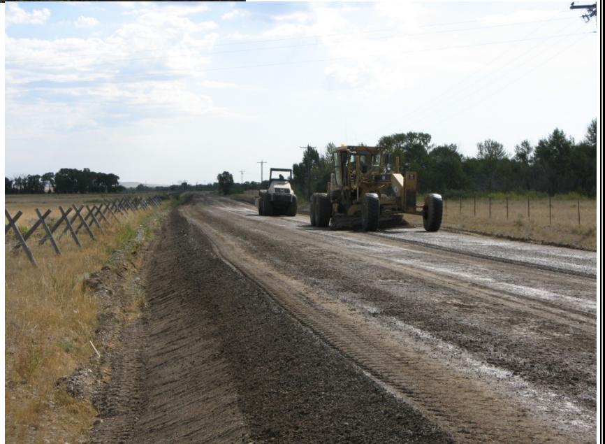
Finishing the roadbed in preparation for crushed aggregate base
