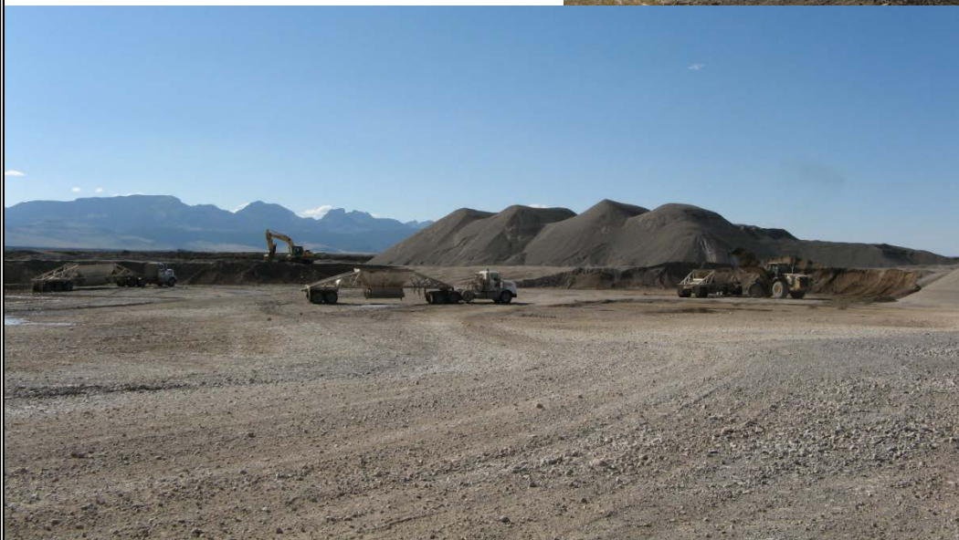
Aggregate base is shown as the large stockpile in the background
