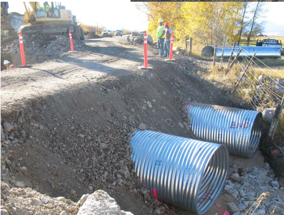
Installation of culvert pipe
