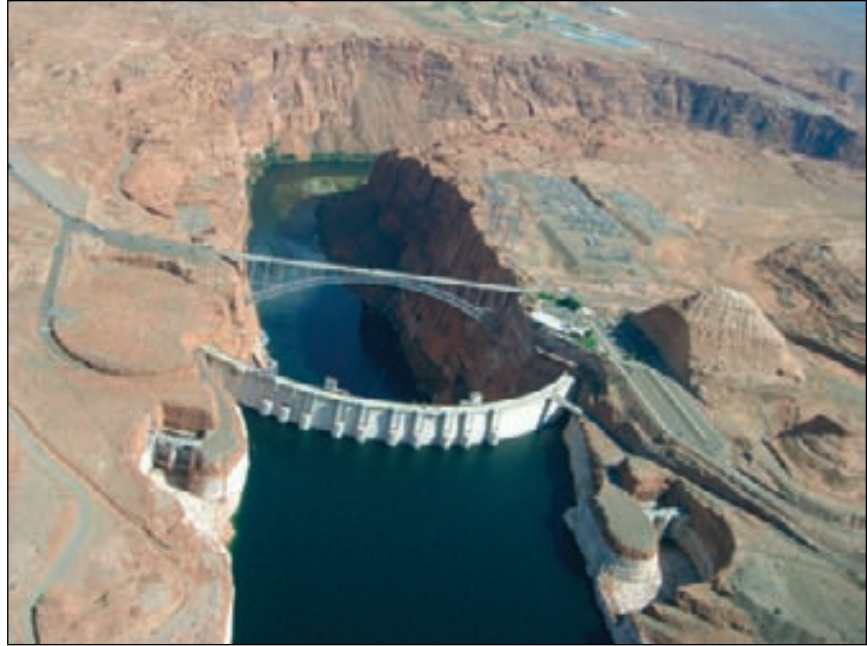
Glen Canyon Dam near Page, Arizona, generates 6 percent of the electricity in Arizona and 13 percent in Utah. (Image from Wikimedia Commons)
