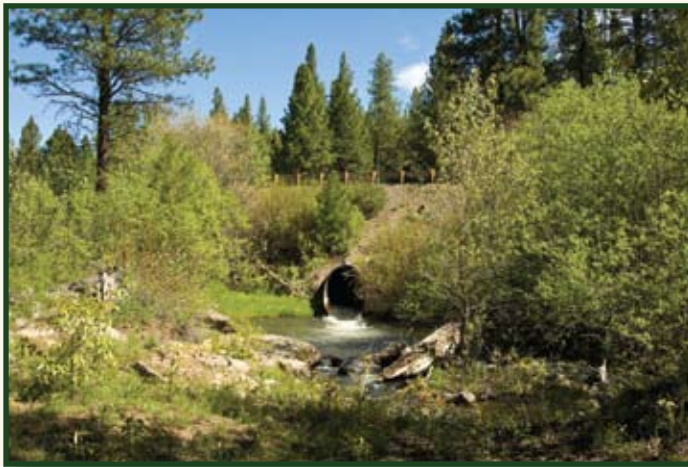
First crossing under current Oregon State Hwy 140 (FH 30)
