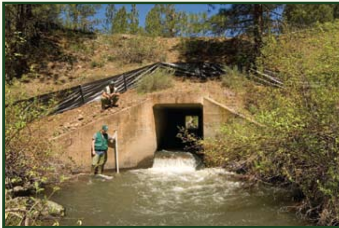
Second crossing under old highway grade
