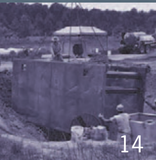
Improving SRS through infrastructure and engineering
