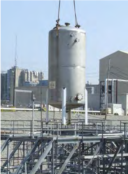
Figure 3.3-9: New Center Riser Cover Being Lowered onto Tank 19
