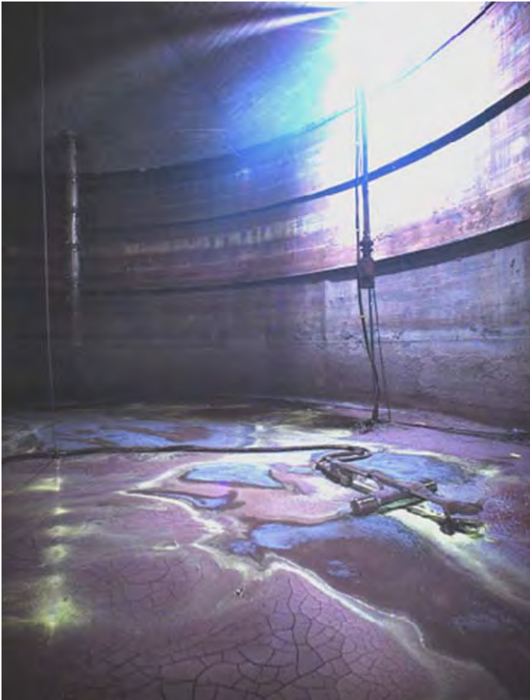
Figure 9.0-3: Tank 18 after Completion of Mantis Operations
