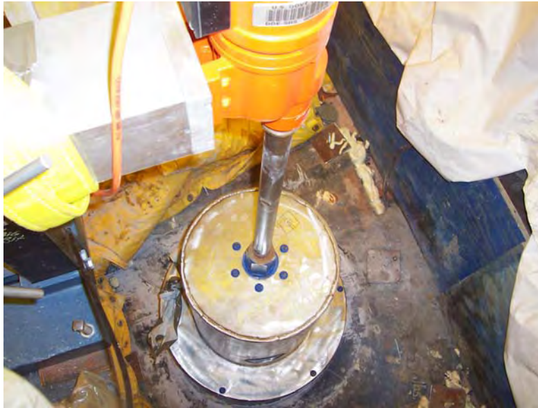
Figure 3.3-15: Core Drilling of New Mechanical Cleaning Riser in Tank 18
