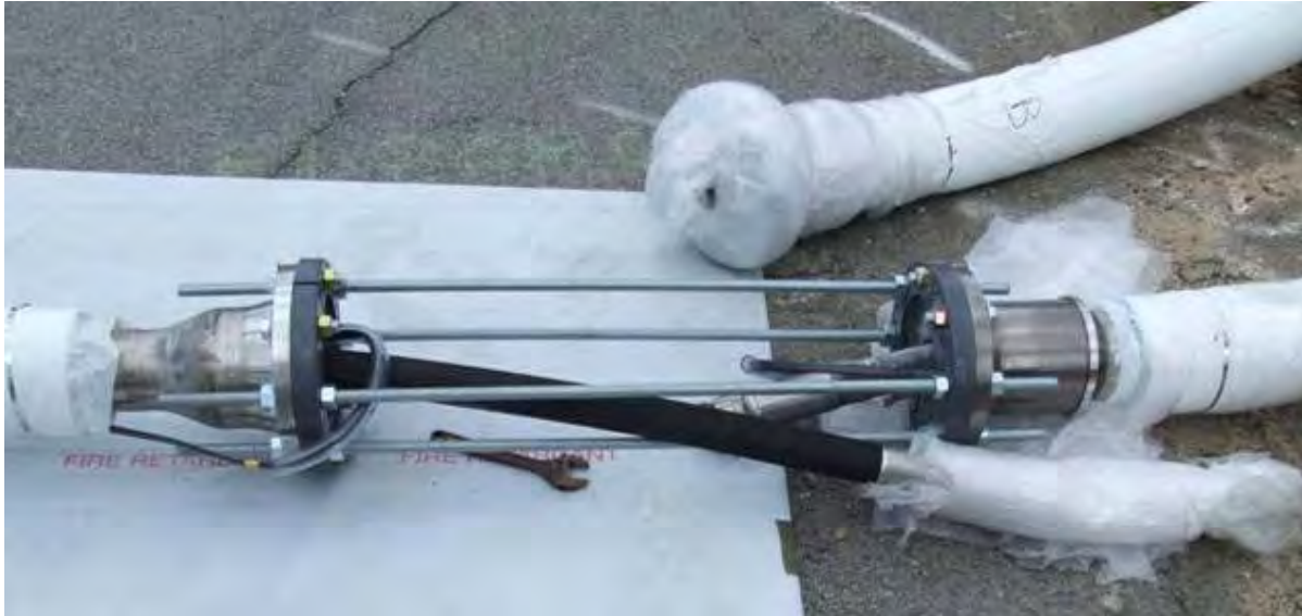
Figure 3.3-5: LDB Location in Hose-In-Hose Transfer Line During Installation
