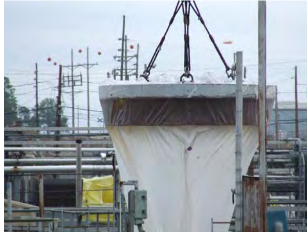
Figure 3.3-8: Removal of the Existing Tank 19 Center Riser Plug
