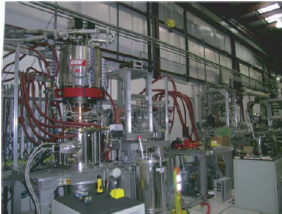
First replacement gyrotron installed in refurbished "socket" and started up
