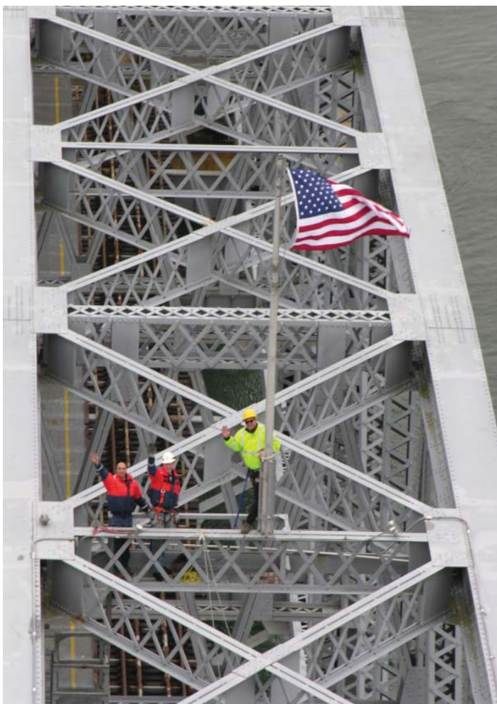
Corps' employees Randy Mello, Ryan Jones, and Richard Patterson replanted the American flag on top of the Cape Cod Canal Railroad Bridge May 17, 2007.
