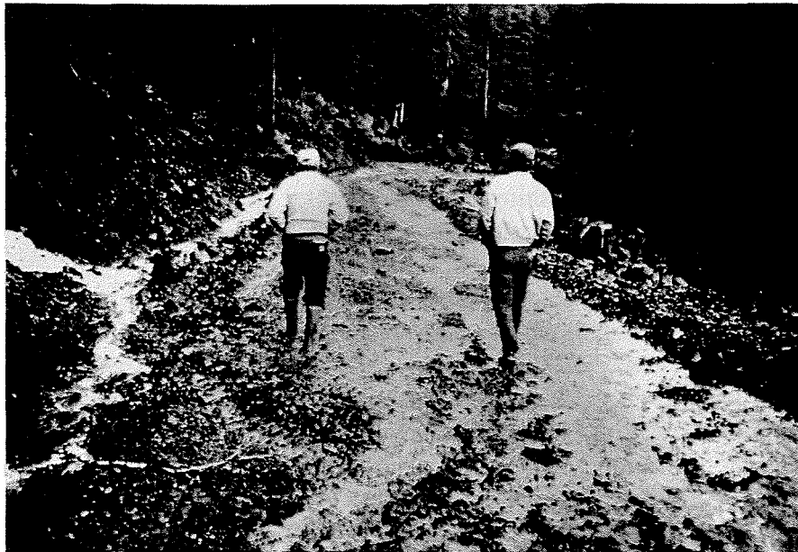
Figure 5.4. Surface runoff being intercepted by a logging road and flowing down the road's ditch after heavy rain in southeast Alaska. (Photo by B. Baker.)
