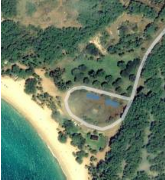
Figure 3-10. IMBY – Hulopoe' Park parking lot
