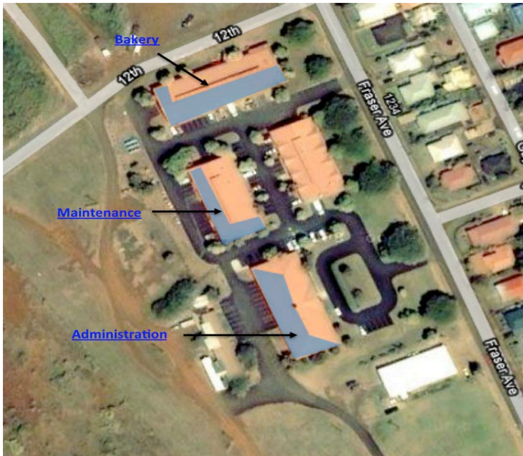
Figure 3-6. IMBY aerial view of the Castle & Cooke central services buildings
