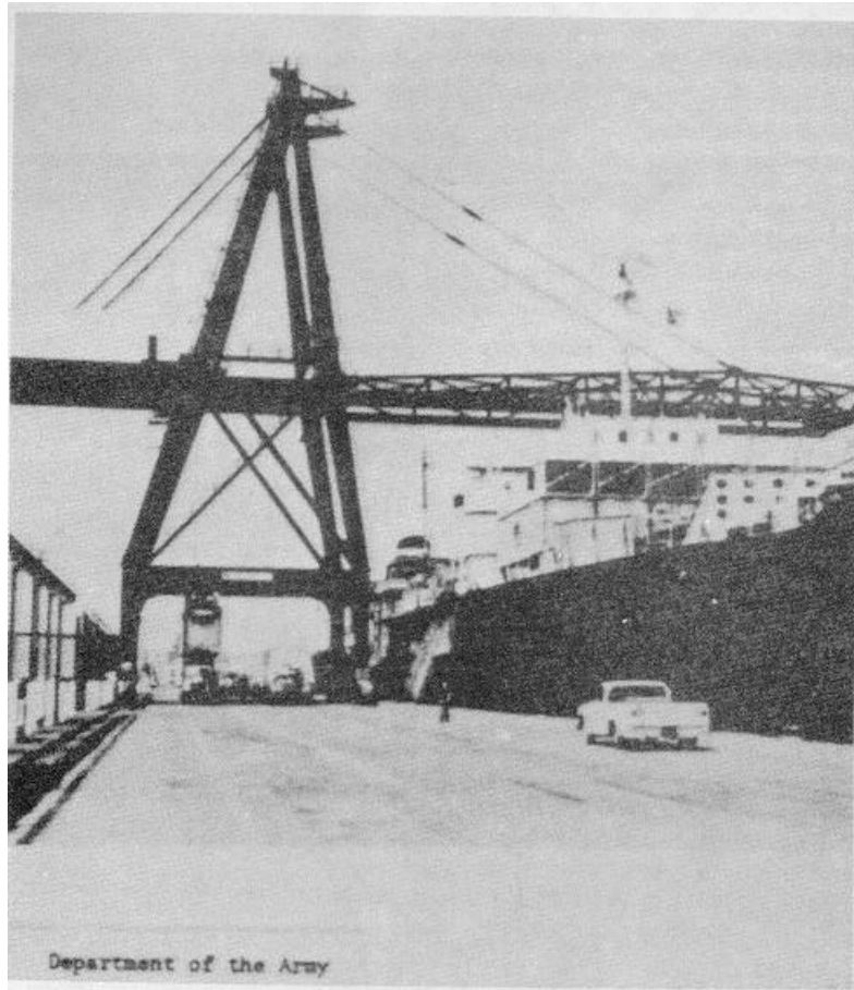
Figure 12-3. Typical rail-mounted gantry crane.
