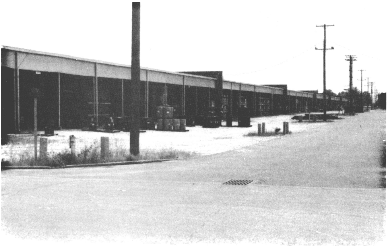
Figure 4-1. Storage shed with floor at road level.
