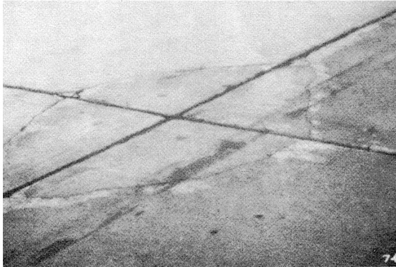
Figure A-70. Low severity corner break, case 2.
