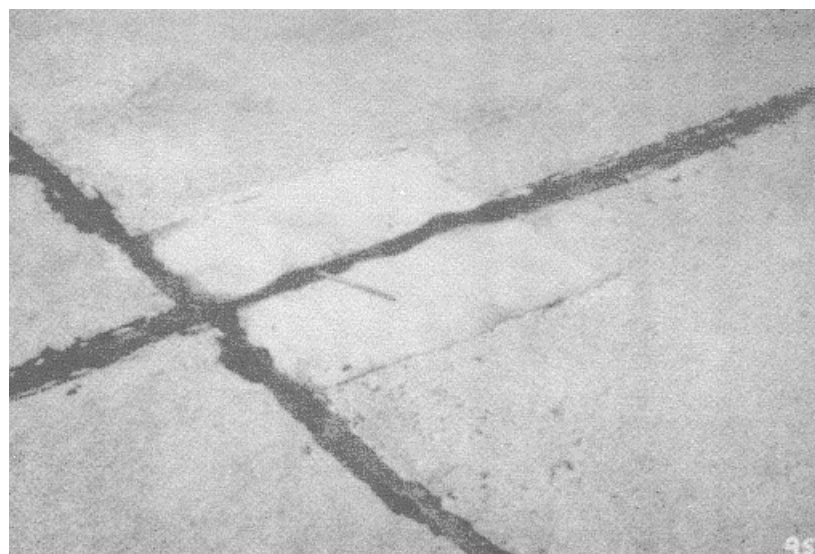
Figure A-92. Low severity small patch, case 2.
