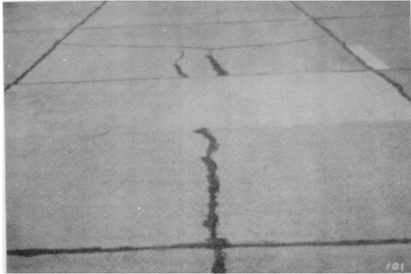
Figure A-97. Low severity patch, case 2.
