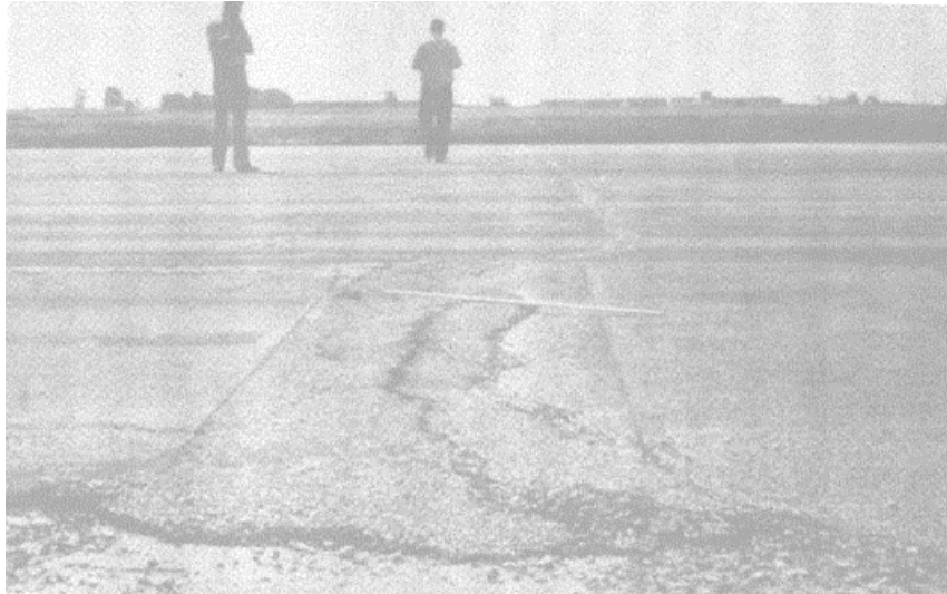
Figure A-65. High severity swell.
