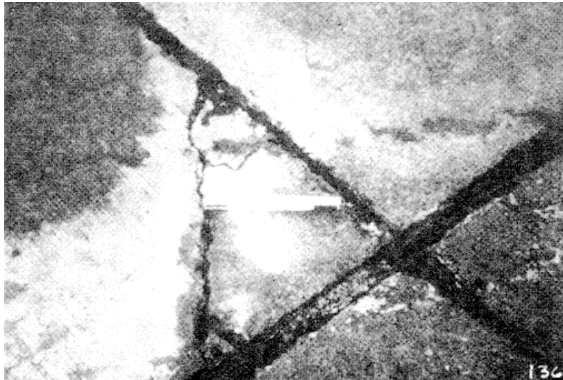
Figure A-132. Medium severity corner spay case 1
