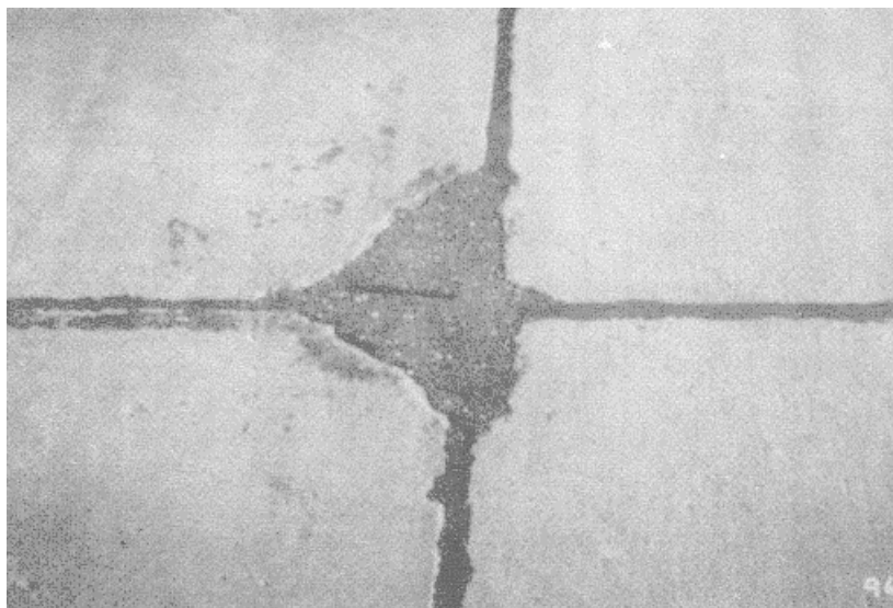
Figure A-91. Low severity small patch, case 1.
