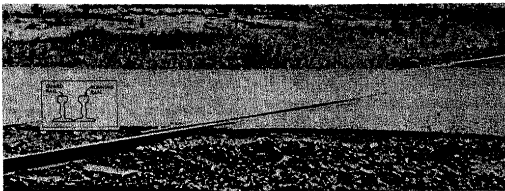
Figure 4-13. Used rail flangeway guard.
