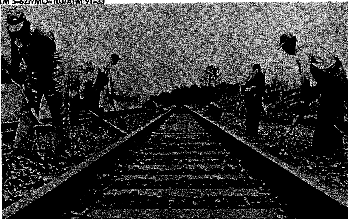
Figure 3-6. Hand-placing ballast after mechanical distribution.
