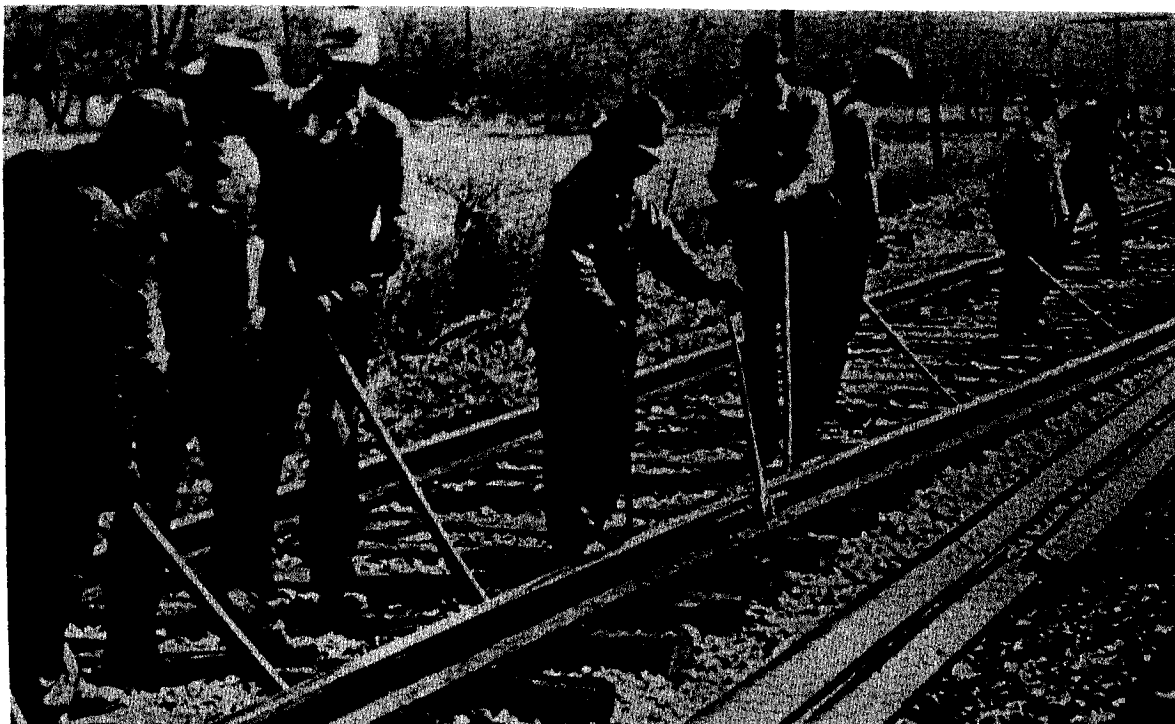
Figure 3-36. Rail being lined out.
