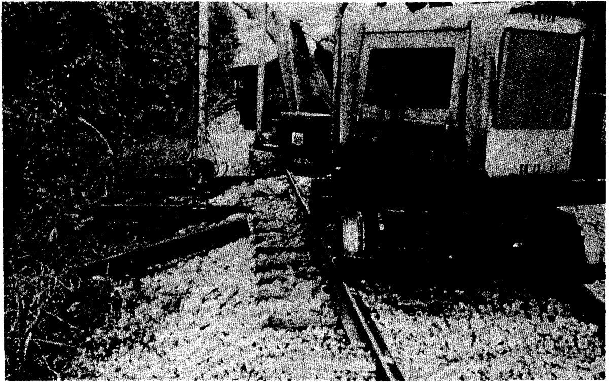
Figure 3-15. Installing ties with a tie crane.
