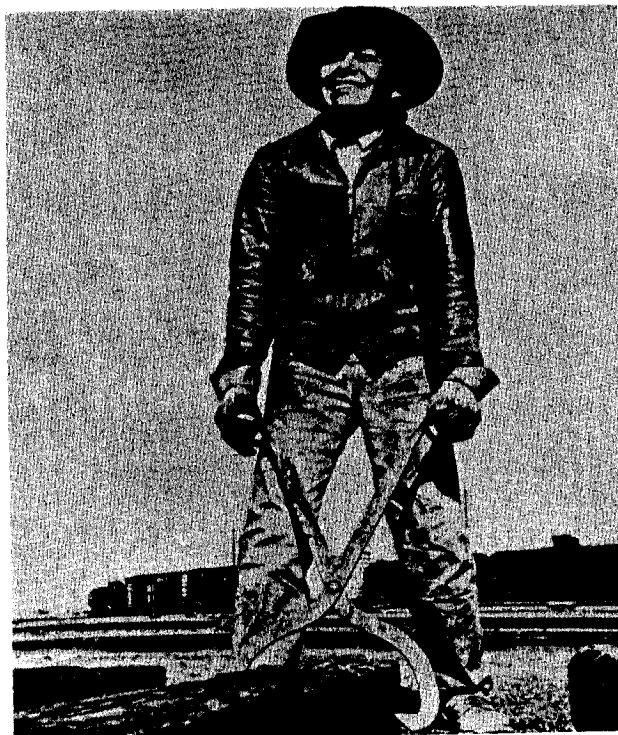
Figure 3-16. Handling treated wood ties.
