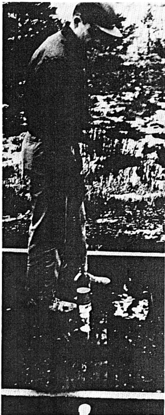
Figure 3-20. Spot marking ties for removal.
