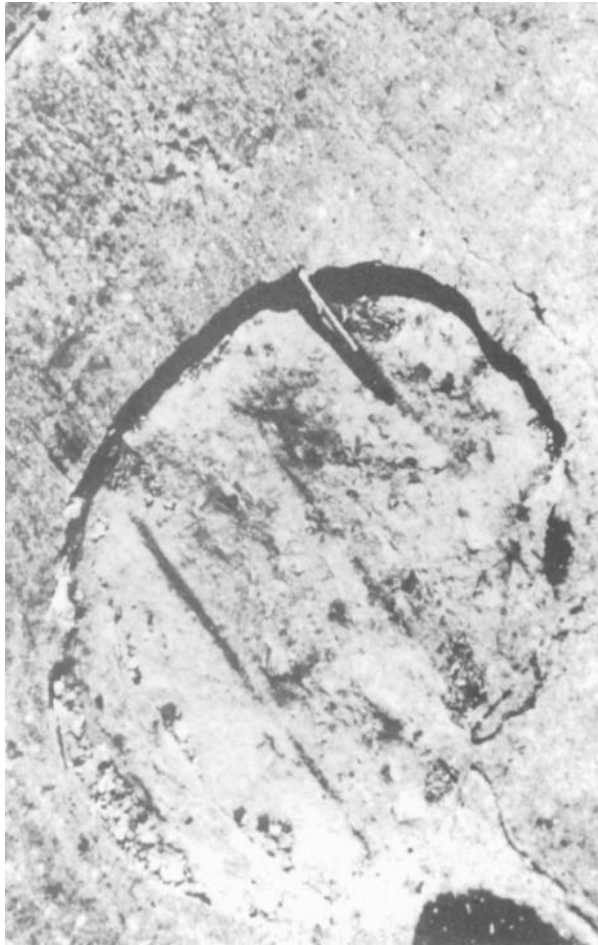
Figure 5-8. Large spall.
