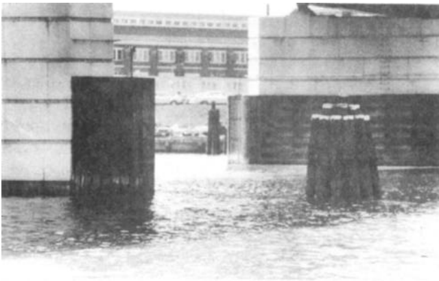
Figure 3-18. Timber pile cluster dolphins and timber fenders.
