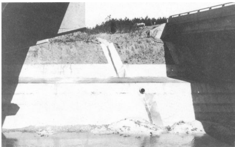
Figure 5-38. Concrete slope protection.
