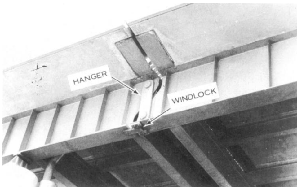
Figure 3-14. Pin and hanger connection.
