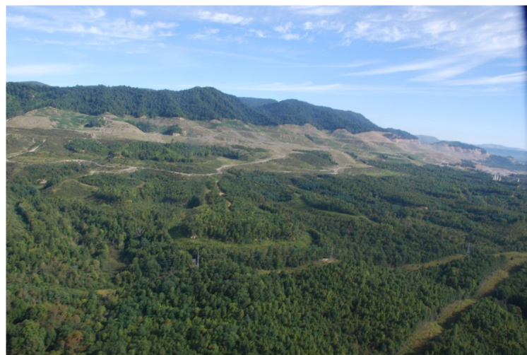
Reclaimed no-cost AML project along the contour through the center: A native forest is rapidly establishing to a point where it is difficult to distinguish the AML project from the adjacent forest.
