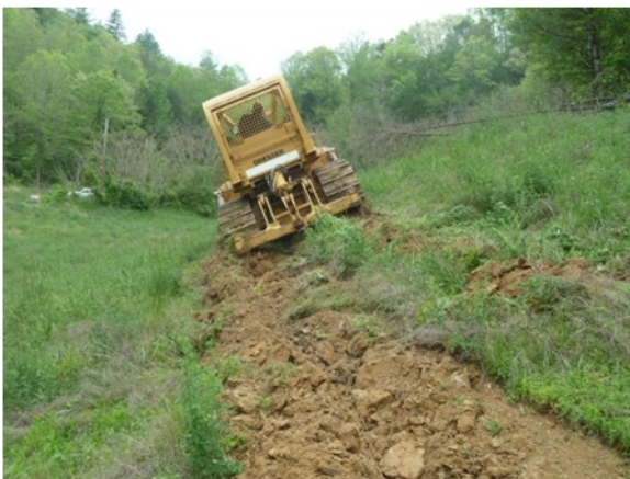
Duane's Trucking and Excavating ripped the site.
