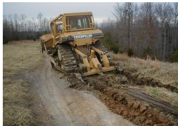
Figure 2. A dozer is ripping to loosen soils and produce soil conditions favorable to successful reforestation in a former roadway.
