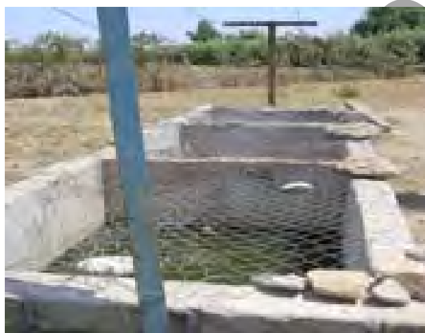
Figure 8-1: Evaporation Tank in Zambia
