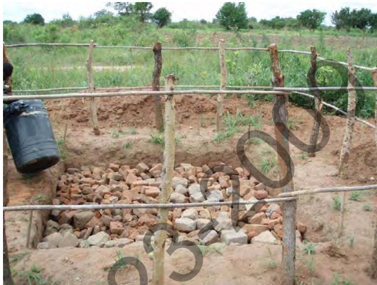
A soak pit that is guarded to prevent the entry of unauthorized persons or domestic animals [Photo: RTI]
