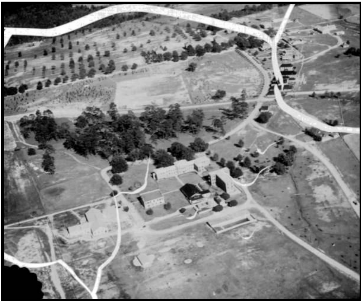
Figure 9. Picture of north department. The road going north to Boot Hill Cemetery is positioned on the East side of the dining hall. Digital image found via the Florida Memory Project, Image Number LC397, original transparency damaged.
