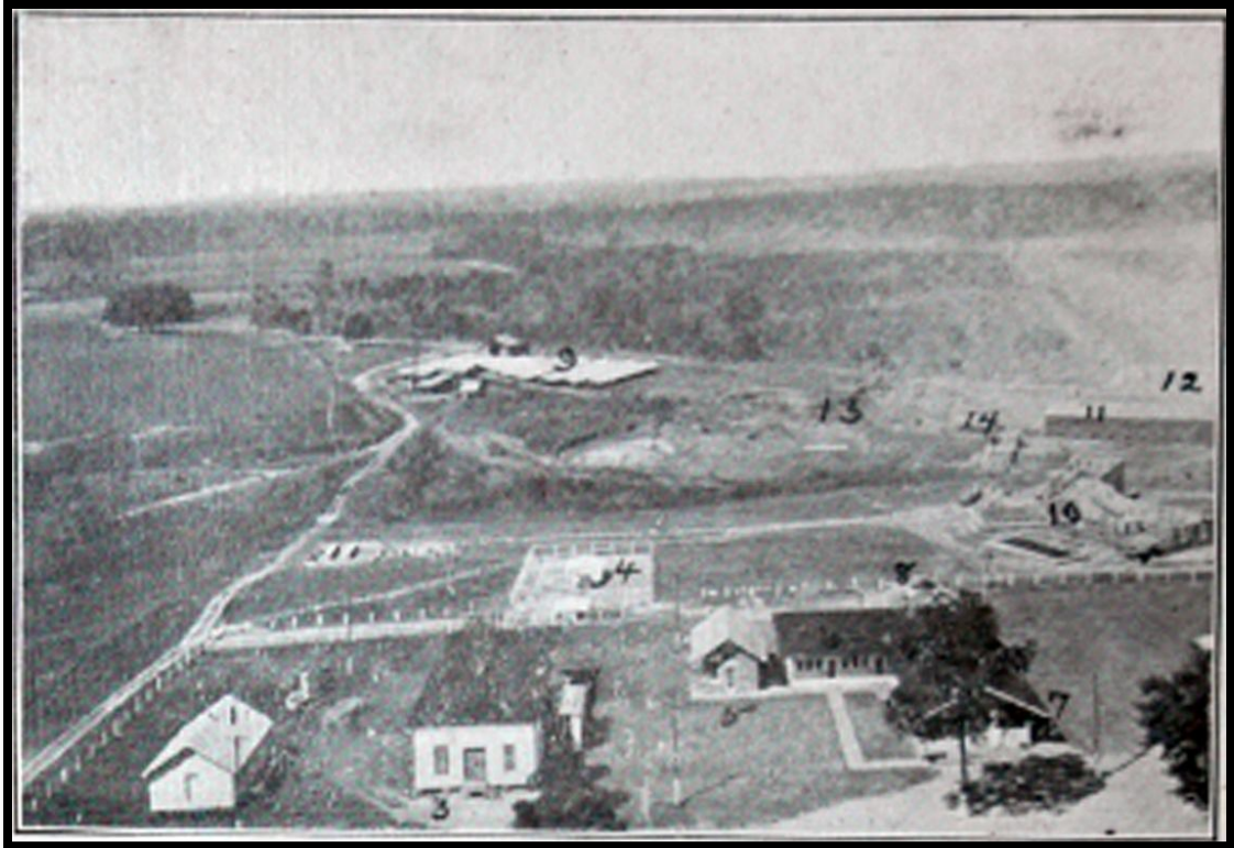
Figure 3. Overview of southern end of south school, illustrating the brick making plant in the background (#9). Image originally published in The Light v. 3, no. 1.
