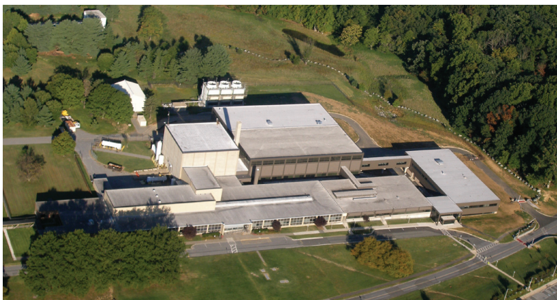
NCNR, including expansion buildings, as seen from the air, Sept. 18, 2010.
