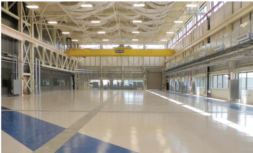
FIGURE 2: – Inside the recently completed guide hall extension. As part of the second construction phase, the dividing wall (shown on the left) between the existing guide hall and the extension will be removed.
