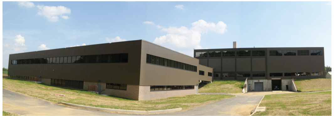
FIGURE 1: Panoramic view showing the completed TSB (foreground, left side,) with a new walkway connecting to the guide hall in the back. The guide hall extension (slightly different wall pattern) can be seen on the right-hand side.
