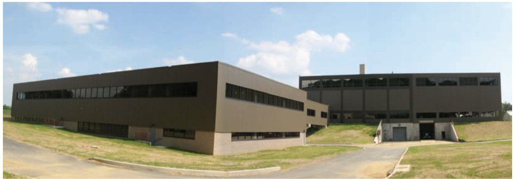
FIGURE 1: Panoramic view showing the completed TSB (foreground, left side,) with a new walkway connecting to the guide hall in the back. The guide hall extension (slightly different wall pattern) can be seen on the right-hand side.
