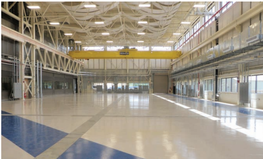
FIGURE 2: – Inside the recently completed guide hall extension. As part of the second construction phase, the dividing wall (shown on the left) between the existing guide hall and the extension will be removed.
