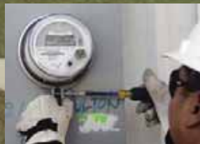
Rod Valencia installs a smart meter for CenterPoint Energy, in Houston, Texas. The utility company, which serves 2.2 million customers in the metropolitan Houston area, expects to spend $1 billion over five years on smart grid and hopes it will pay for itself in efficiency savings. (AP Photo/Pat Sullivan)
