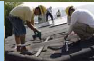
Installers Arin Gharibian and Hayk Mkrtchyan, employees of California Green Design, assemble supports for solar electrical panels on the roof of a home in Glendale, California. (AP Photo/Reed Saxon)
