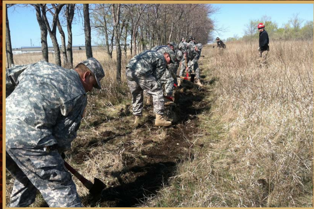
Right, Soldiers of the 816th Engineer Company and the 957th Engineer Company (Multi-Role Bridge) repaired flood damage to roads at Kimball Bottoms, south of Bismarck, N.D., April 21. The units graded roads, filled washed out areas, removed sand deposits and moved fallen trees. The 957th will train with their float bridge at Kimball Bottoms later this month.
