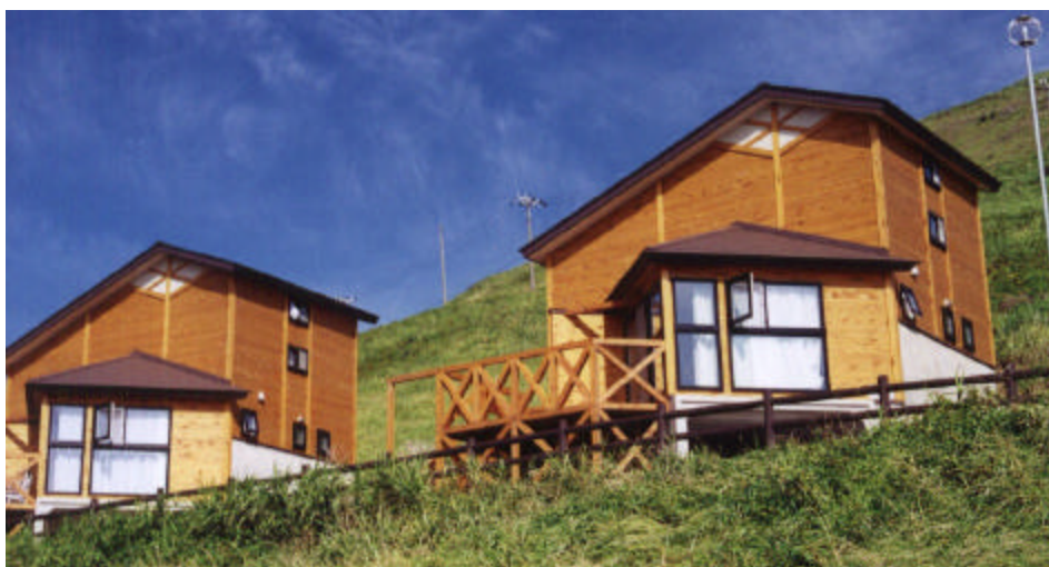
[Above] Newly constructed bungalows at Tappizaki Campground offer all the comforts of home, including showers and full bathroom, kitchen, TV etc.
