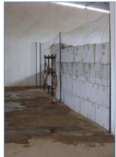
Floor in this storage facility is wet. This could indicate a problem. Boxes should be stacked on pallets to protect the pesticide from contact with moisture.
