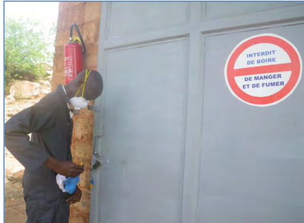
Storage facility with double lock, fire extinguisher, and warning sign
