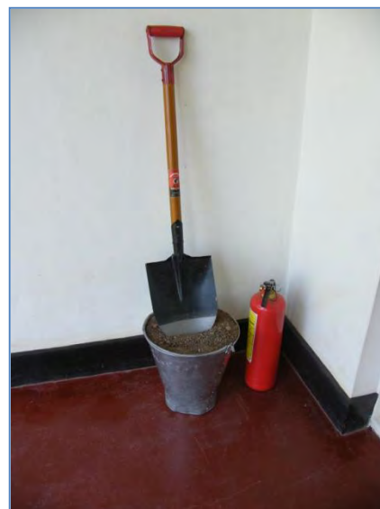
A spill response kit: bucket with sand, shovel and fire extinguisher
