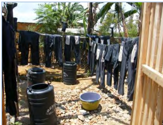
Soak pit with warning sign and secured lockable fencing
