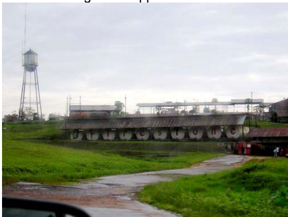
Figure 4. Firestone Plant in Margibi
