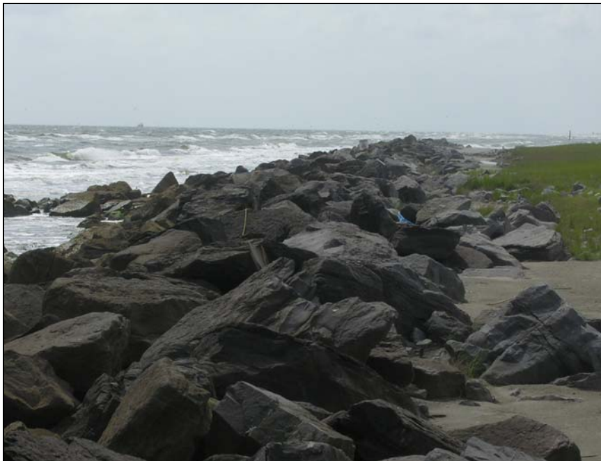
Figure 2-27. Shoreline protection feature located on Timbalier Island
