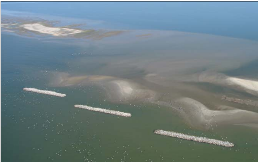
Figure 2-6. Northerly view of existing breakwaters on Raccoon Island
