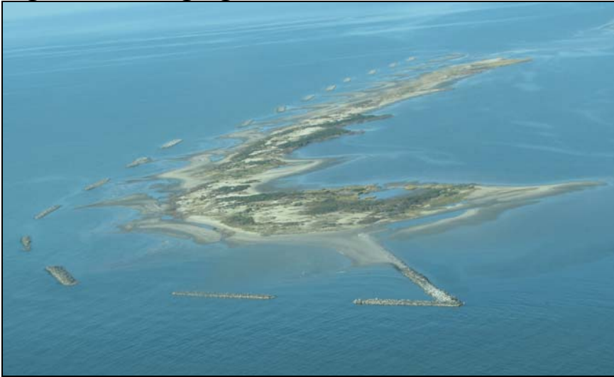
Figure 2-5. Aerial view of existing breakwaters on Raccoon Island
