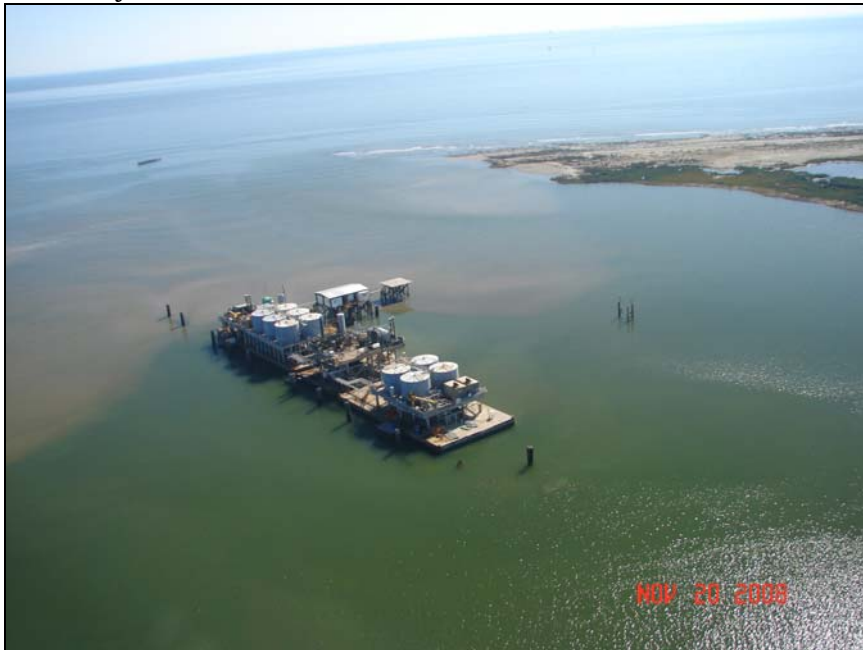
Figure 2-10. Oil and gas facility located east of Whiskey Island
