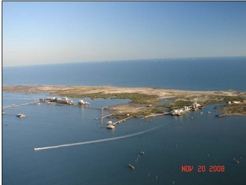
Figure 2-30. View of the oil and gas facilities protected by East Timbalier Island
