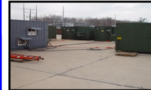
Containerized Maintenance Facility
