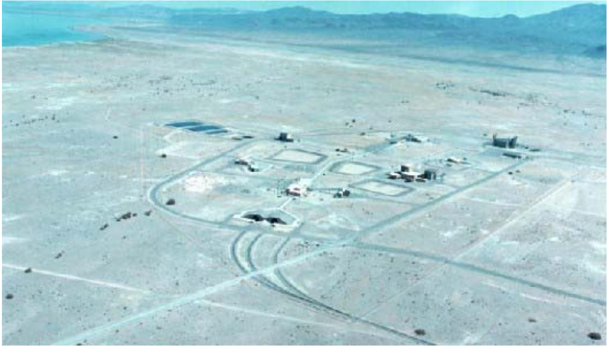
WADF under construction
