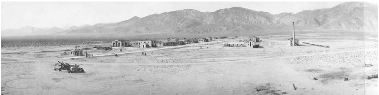
Construction of the Industrial Area, 1930
