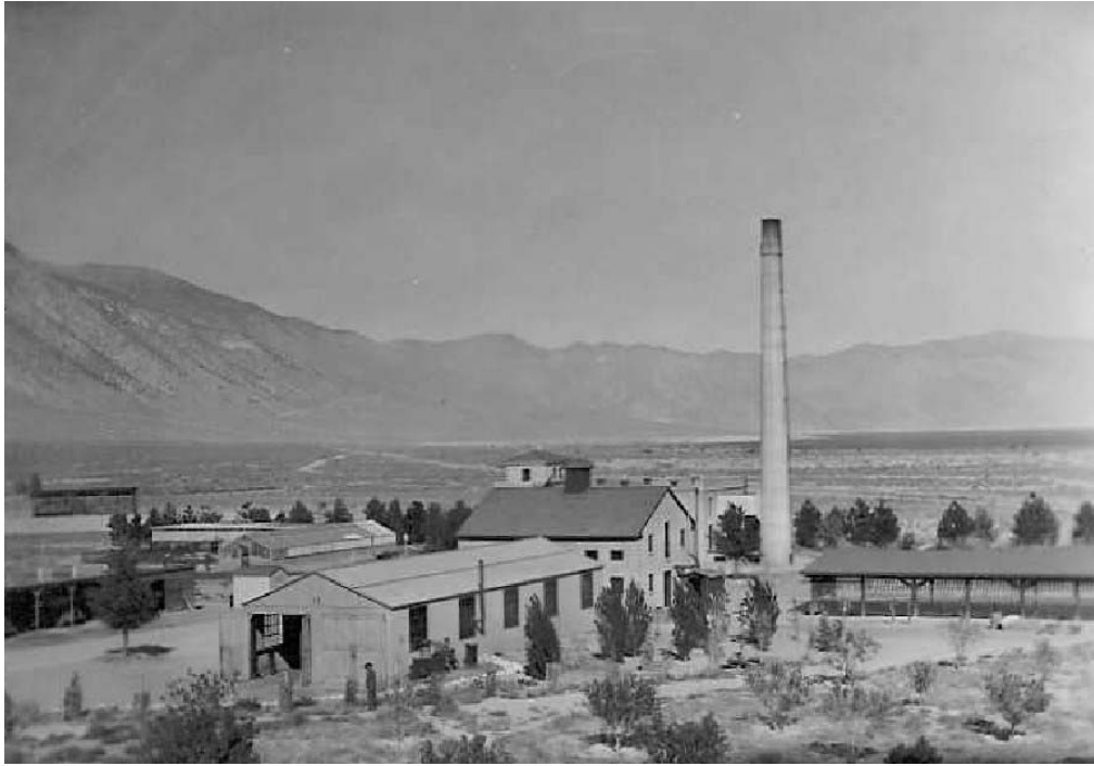
Boiler, Stables, and Green House, 1945
