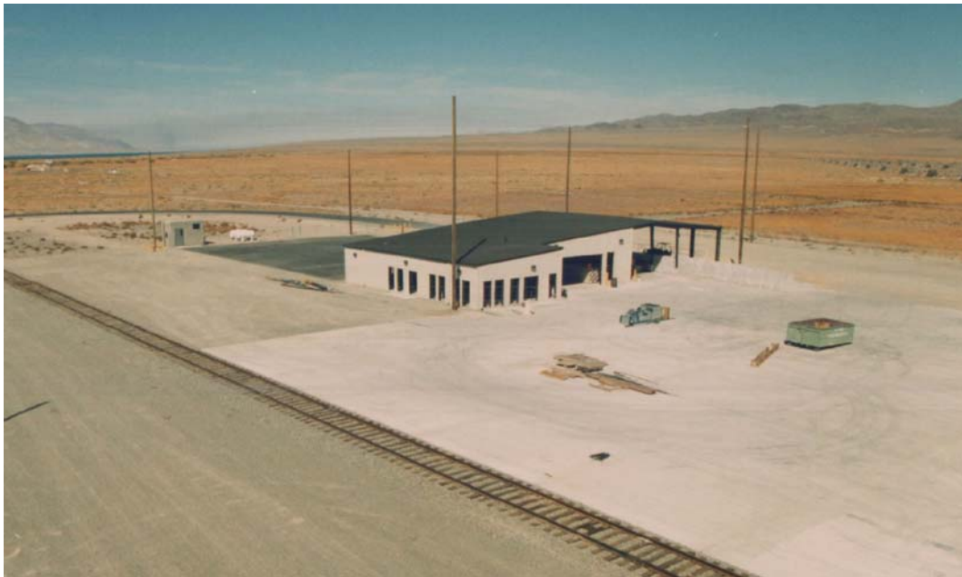
New loadout area
