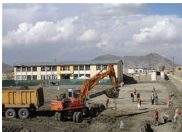
Building a high school in Kabul (source: USAID)
