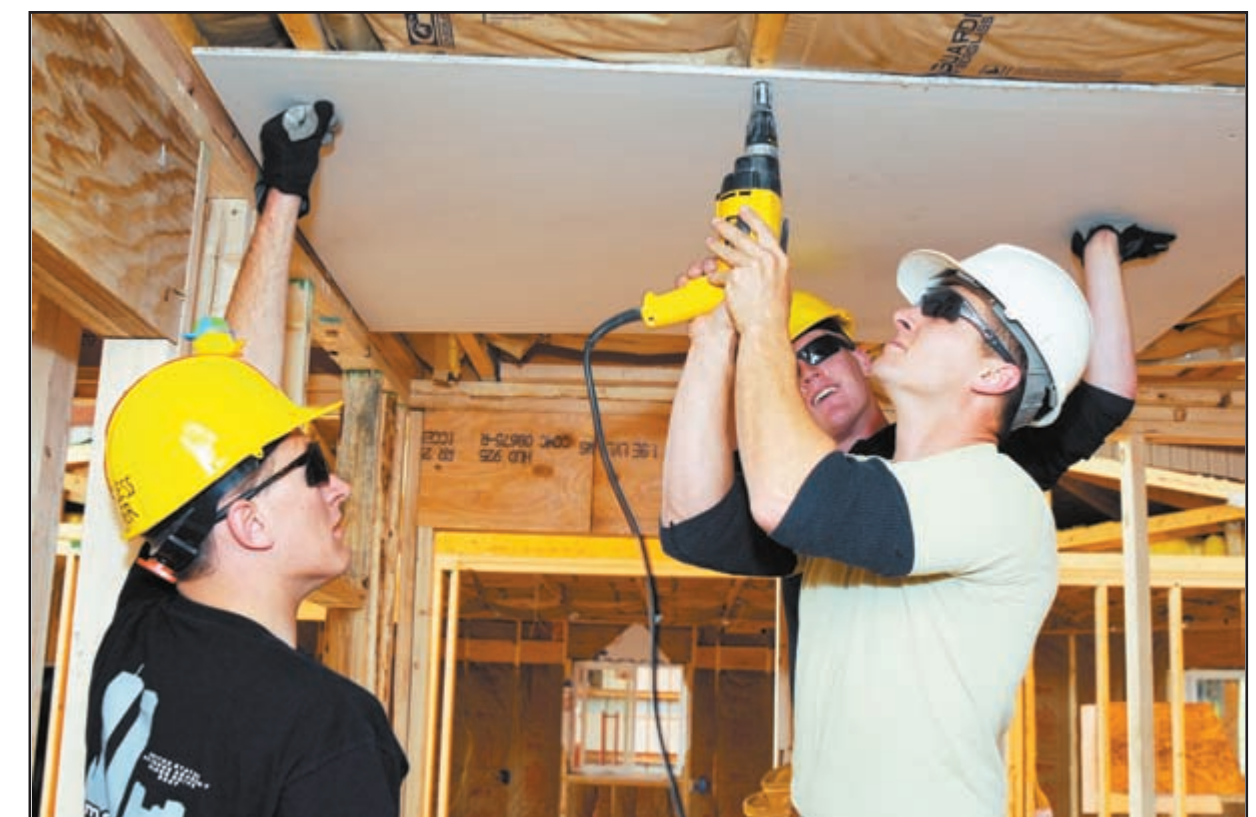
Cadets 1st Class Jon Brateng and Matt Buscemi, along with mentor Tech. Sgt. Denver Long from Whiteman AFB, MO, hang drywall in the wood frame activity.
