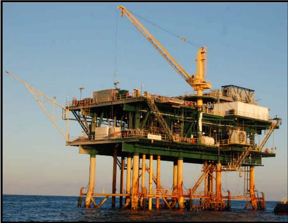
Figure 3 - HI A557 "A" Platform
