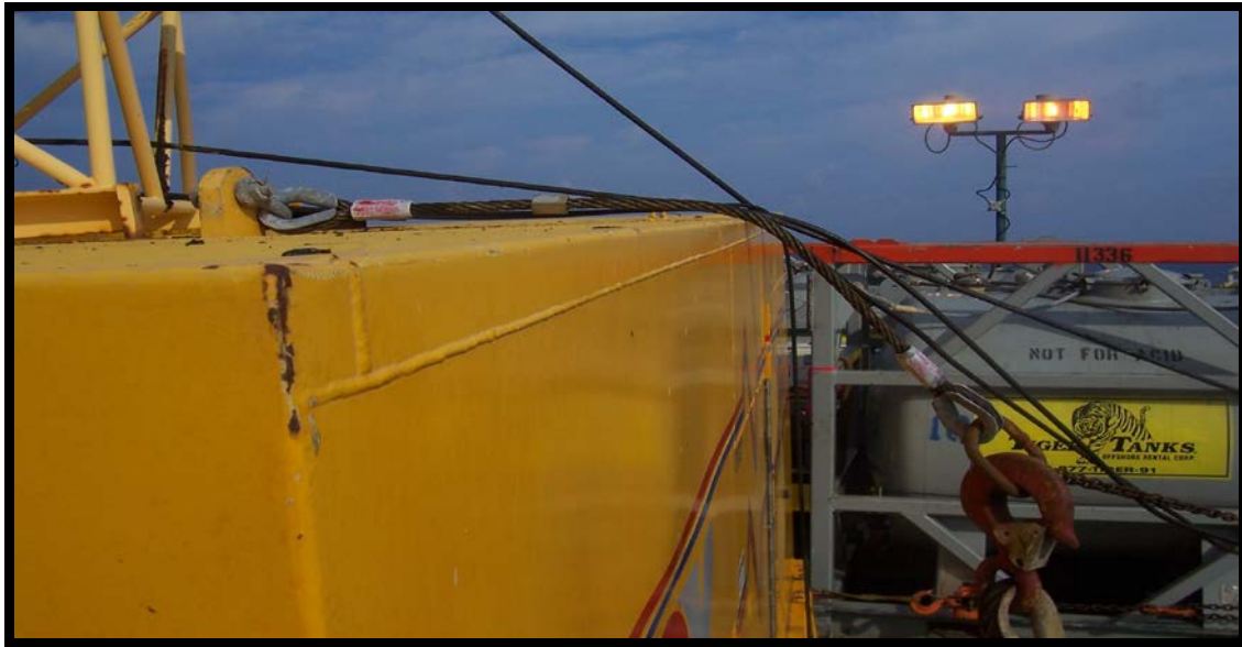
Figure 26 – Stinger hook attached to the generator rigging
