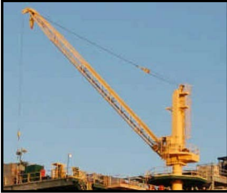
Figure 6 – SeaKing Model 1400 Crane on Platform
