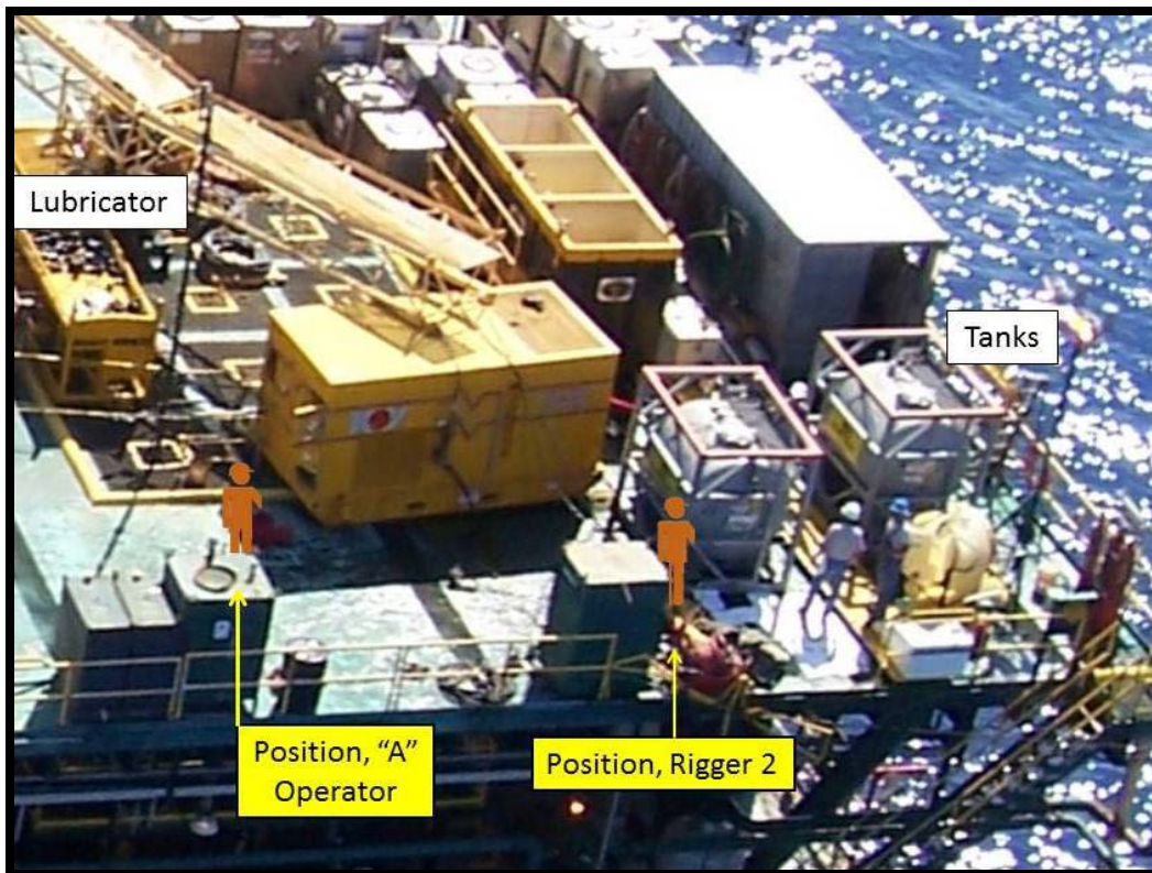
Figure 13 - Position of riggers, equipment
