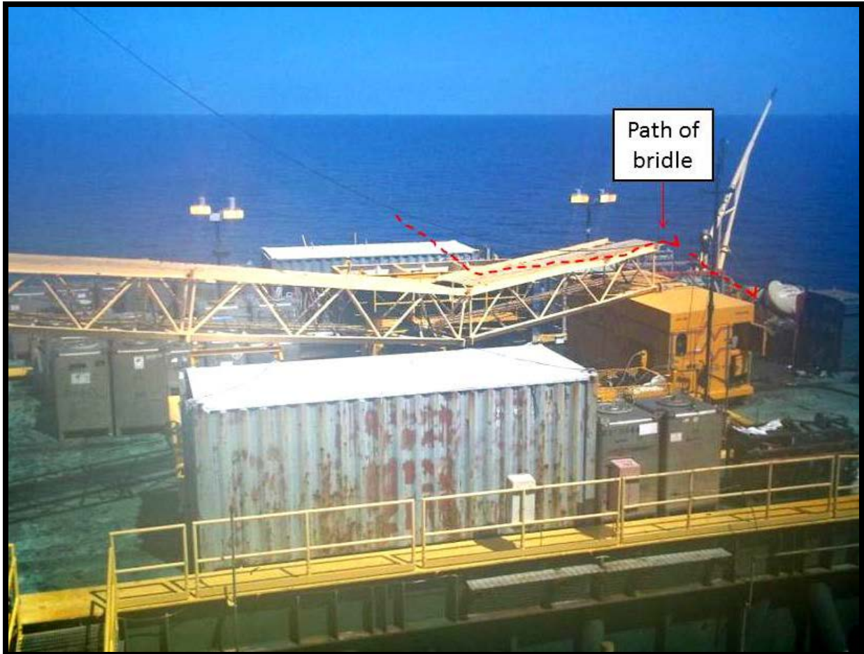
Figure 15 – Separated boom atop the rental generator
