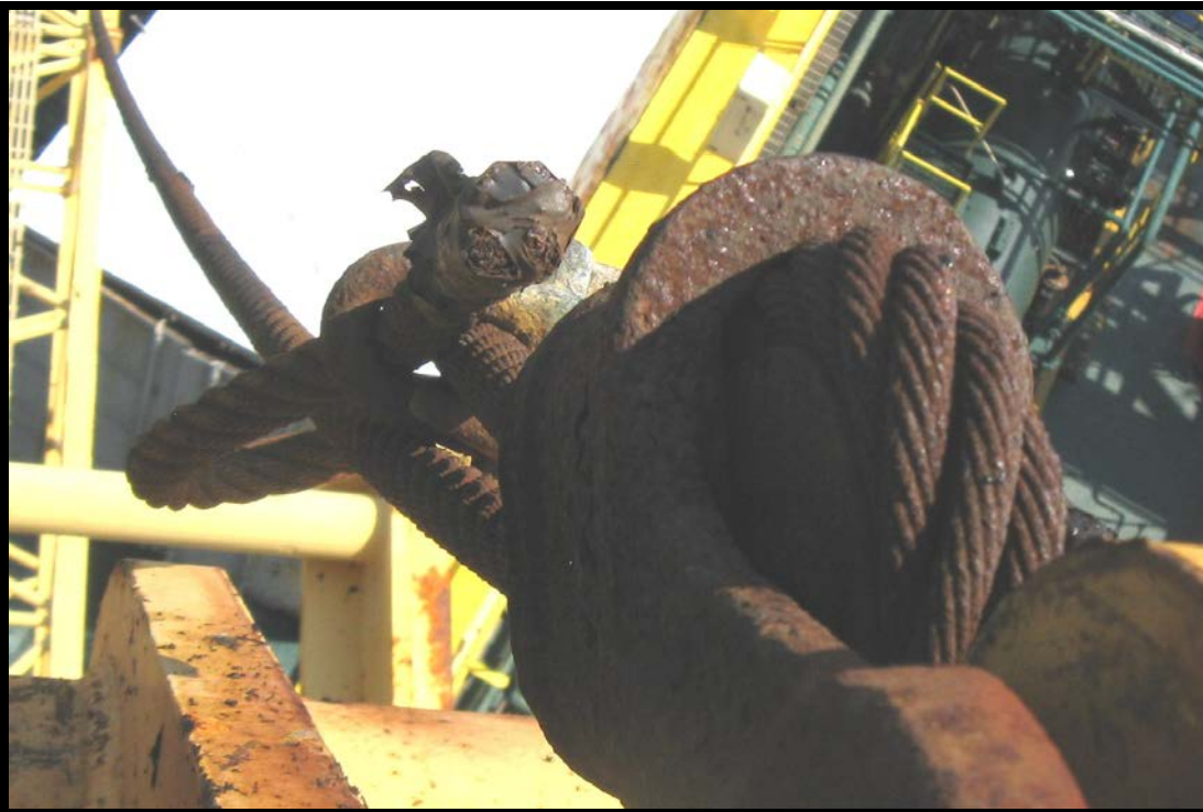
Figure 23 – Corroded boom hoist wire rope, wedge socket, pinned to gantry dead end connection
