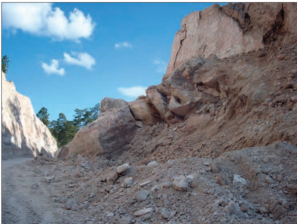
Figure 17: Landslide in CA-5 Section 2, Honduras Transportation Project
