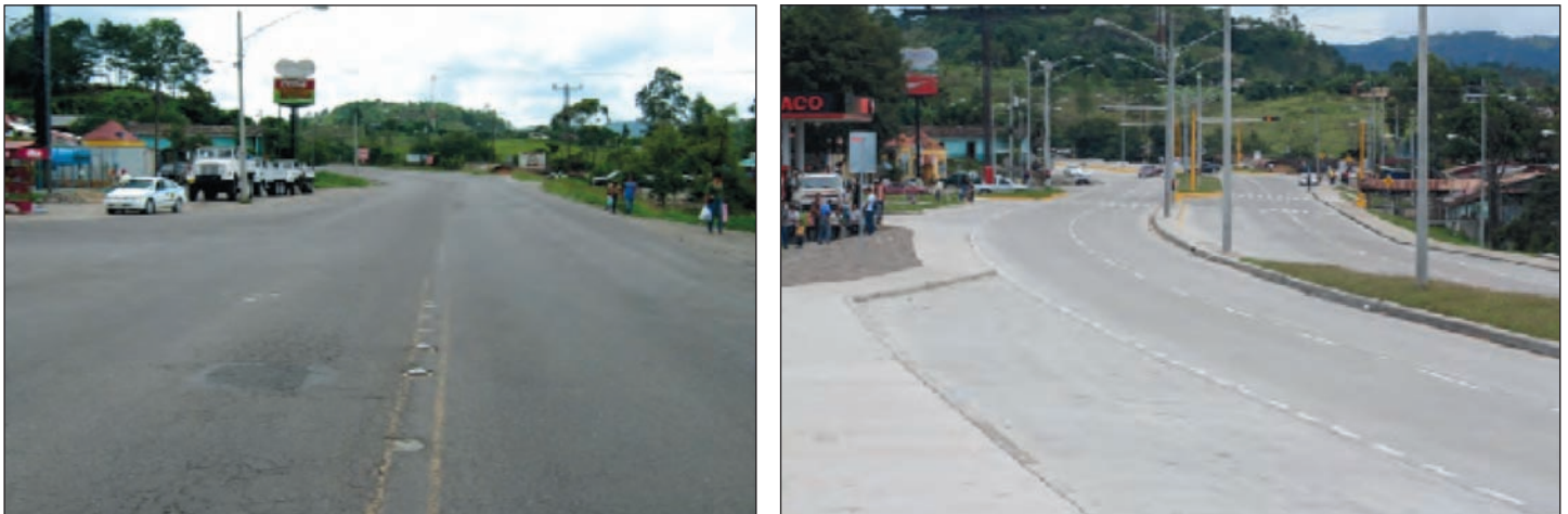
Figure 11: CA-5 Section 4 before and after Reconstruction, Honduras Transportation Project
