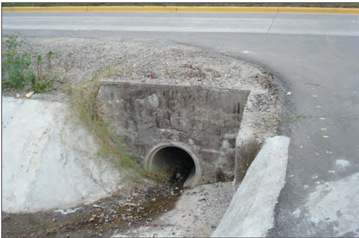
Figure 19: Locations on Completed CA-5 without Traffic Safety Devices, Honduras Transportation Project
