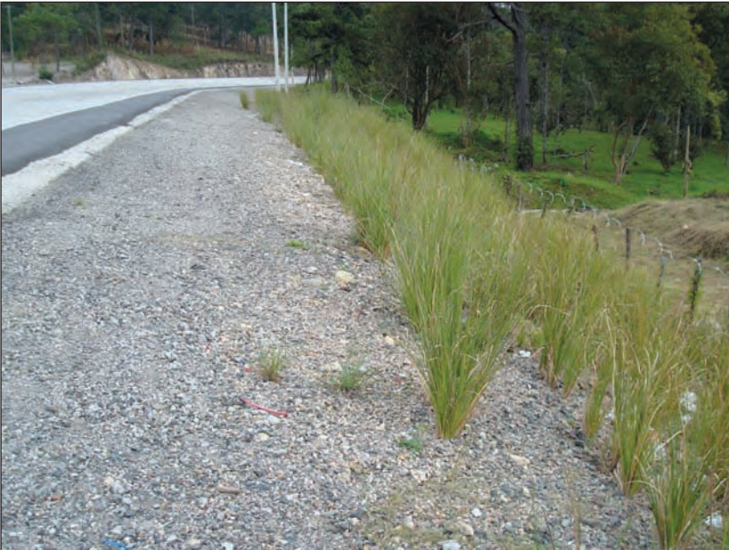
Proper revegetation of fill slopes along CA-5
