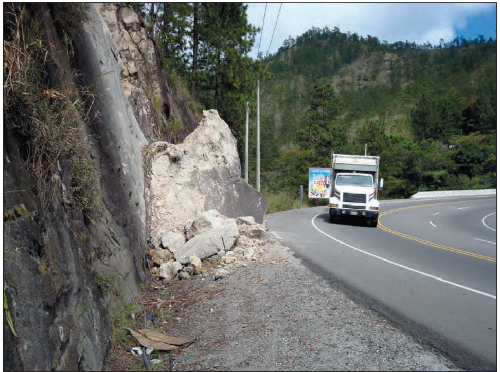
Figure 7: Landslide on CA-5 Section 3 in Honduras
