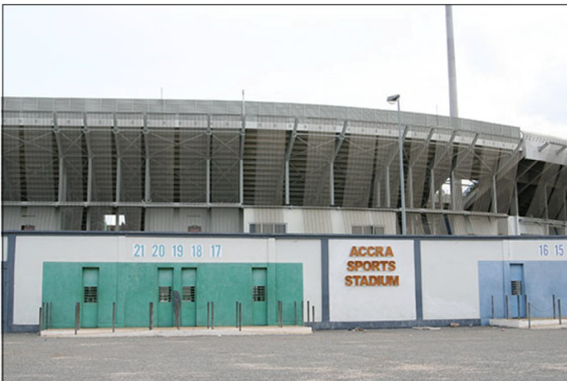
Source: GAO. Accra Sports Stadium, the primary soccer arena in Accra, Ghana, renovated by a Chinese firm for the 2008 Africa Cup of Nations.
