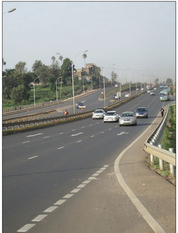
Source: GAO. Nairobi-Thika Highway, built by three Chinese state-owned firms and funded by the African Development Bank and the Chinese government in Kenya.
