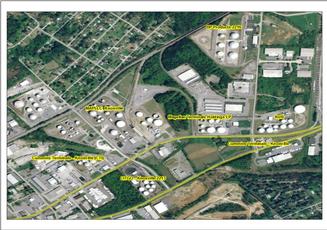
Fig. 62. Terminals around the Knoxville, Tennessee, region.
