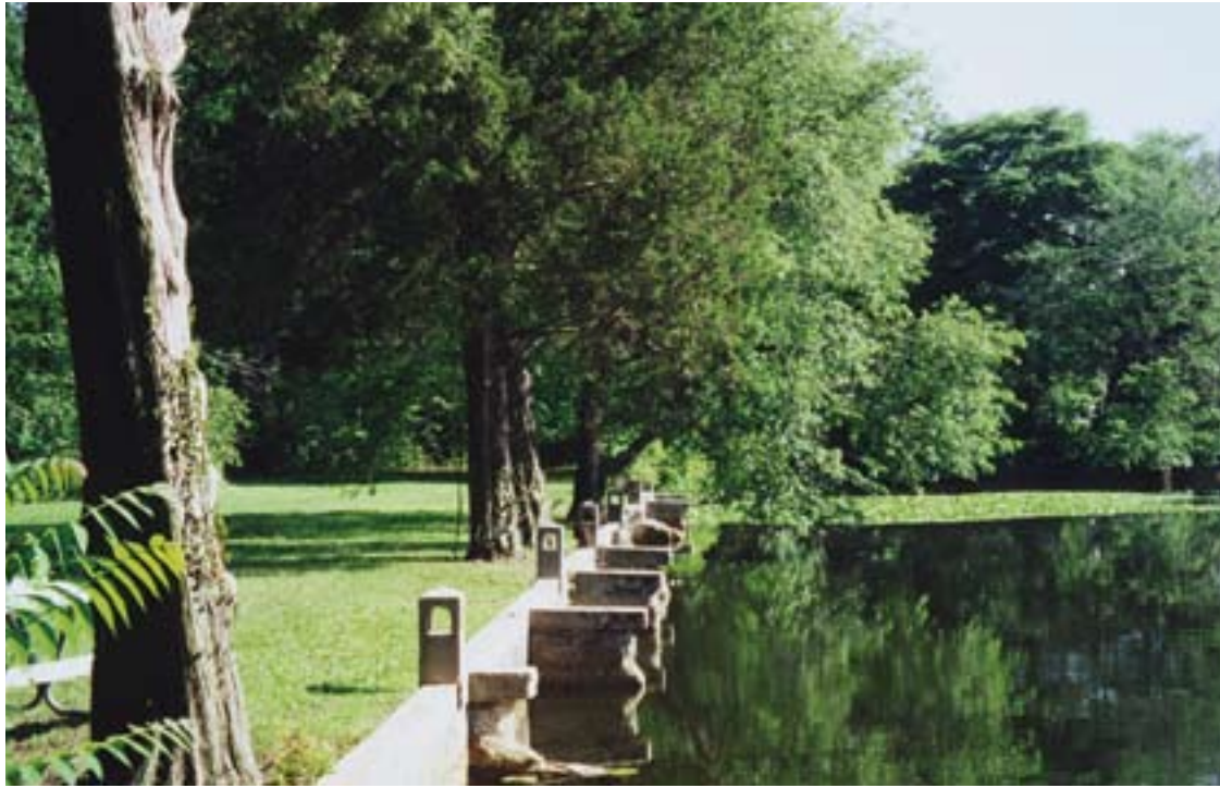
Concrete decorative retaining walls lining the edge of Dr. Stewart's Old Fishing Hole, 1999.
