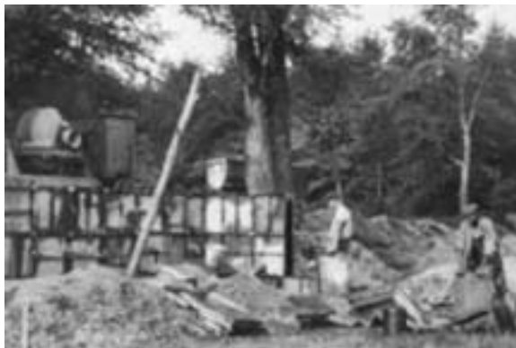
Construction of the concrete retaining wall between Belle Chance and Dr. Stewart's Old Fishing Hole, one of the three spring-fed ponds behind the property, 1920.
