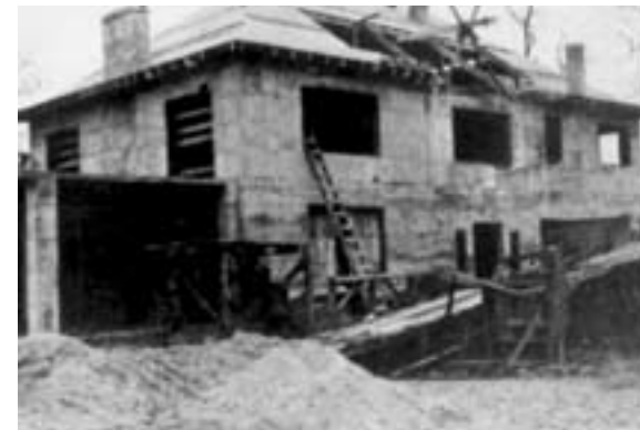
Dr. Stewart's new all-concrete Belle Chance in 1912, under construction and during the summer and autumn. It was one of the first buildings in the area designed to be completely fireproof.
