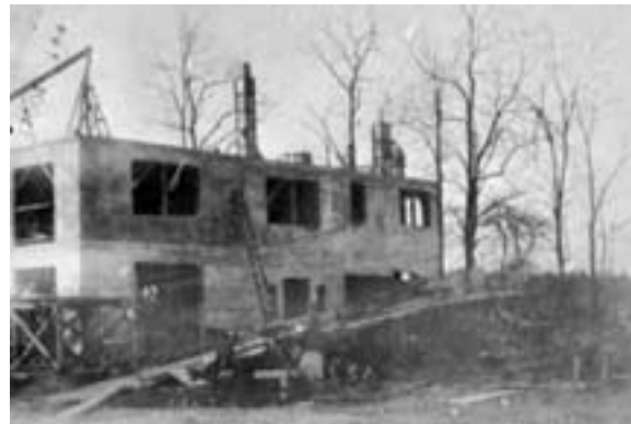
Dr. Stewart's new all-concrete Belle Chance in 1912, under construction and during the summer and autumn. It was one of the first buildings in the area designed to be completely fireproof.
