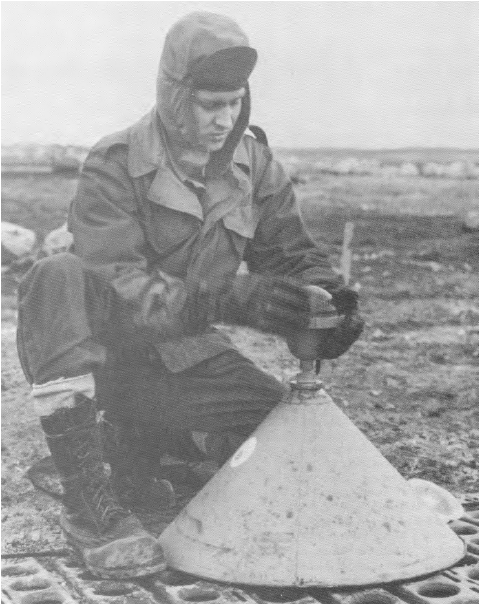
An airport maintenance mechanic checks a landing strip light which enables planes to operate around-the-clock.
