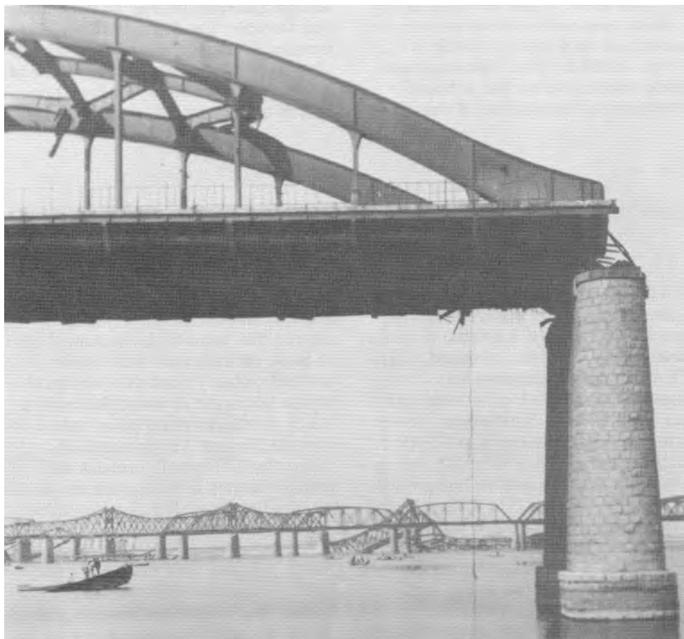
Bridge-busting activities on the Han River.
