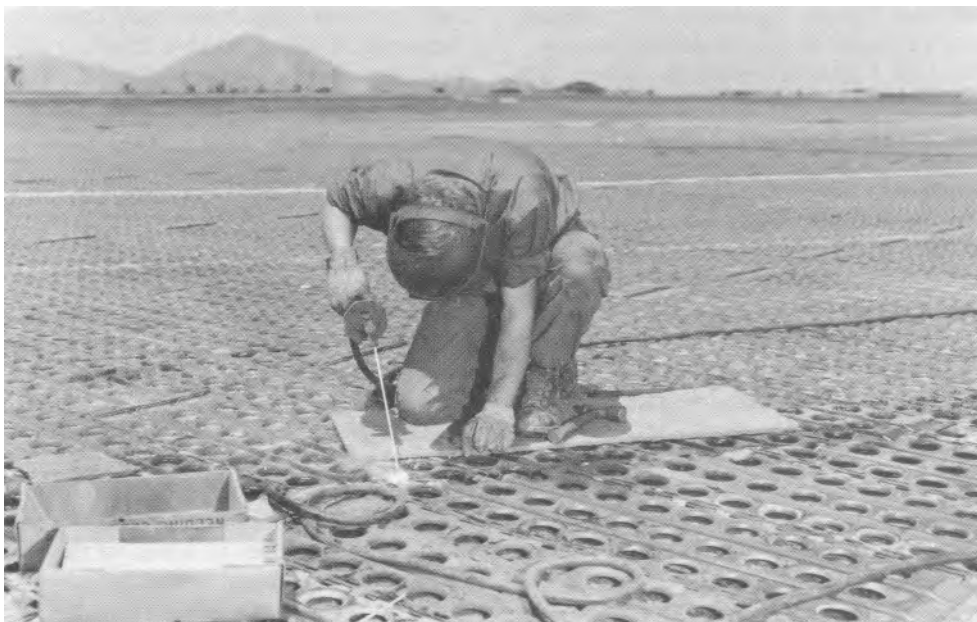
Welding torches were used to repair pierced steel planking.
