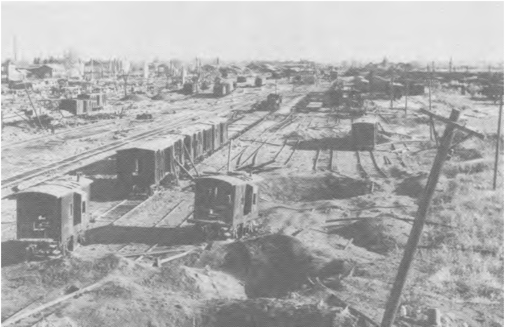
Wreckage of railroad yard at Pyongyang following attacks on the airfields and city.
