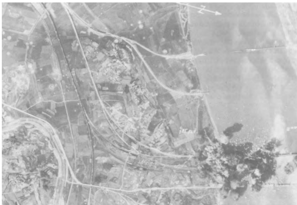
Five rail and highway bridges are knocked out at this rail complex near Sinanju, 4 September 1951.
