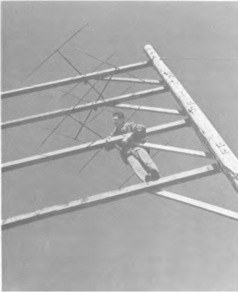
A3C Nick Psairas of the 502d Tactical Control Group adjusts a hilltop radio relay directional antenna to the proper channel.
