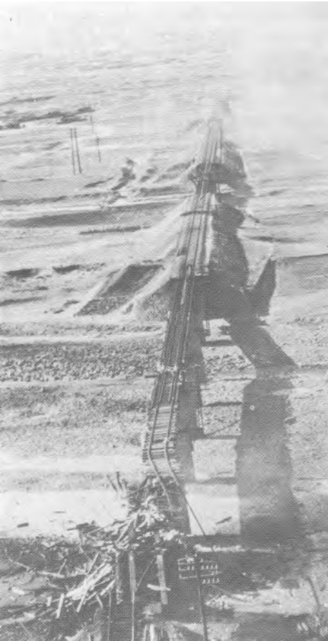
Damaged enemy rail bridge.
