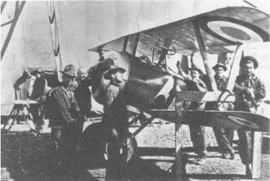
Repairs are made to the wing and strut of a damaged Nieuport 27.
