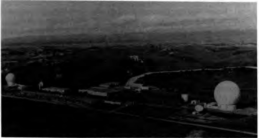
The ground tracking station at Vandenberg AFB. A network of such Air Force ground stations track, command, and control all U.S. military satellites as they orbit the Earth.
