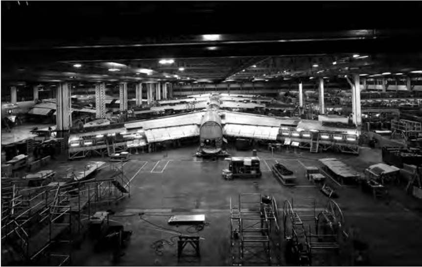
These B-52s are in the final stages of assembly in May 1954.
