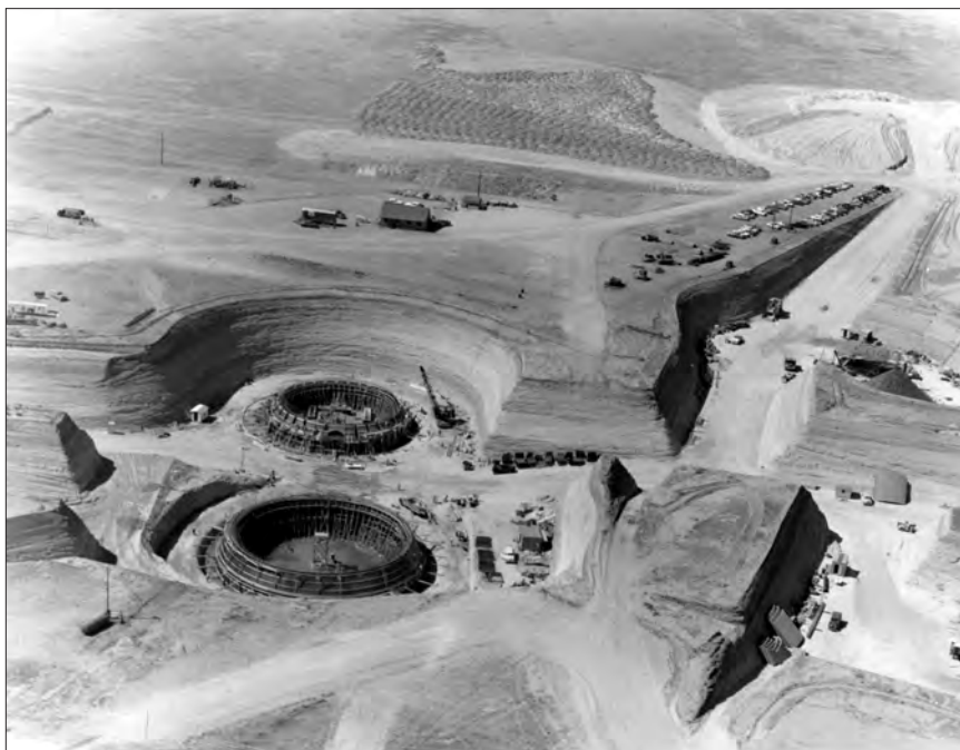
Launcher sites for the Air Force's strategic nuclear weapon, the Titan ICBM, were under construction from the late 1950s through the early 1960s at Lowry AFB near Denver, Colorado.
