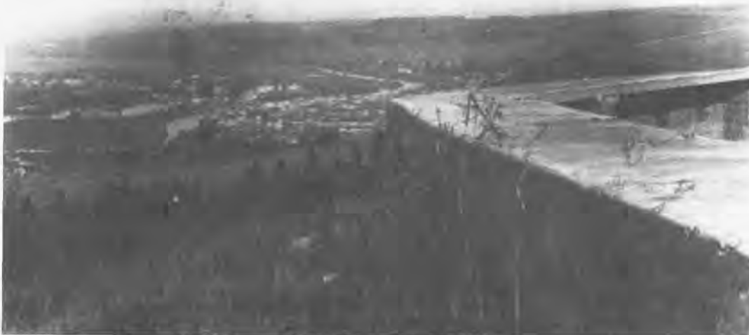
A concrete rampart overlooking St. Mihiel.
