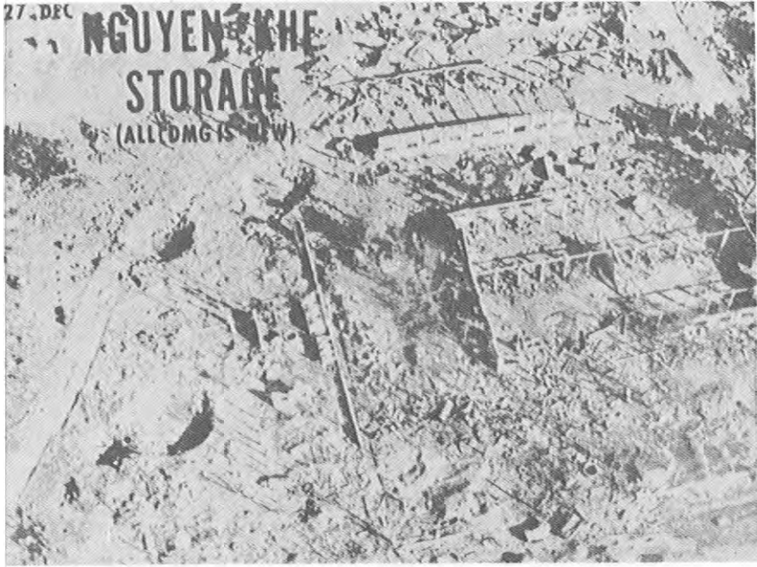
This low altitude photo shows the degree of damage which was characteristic in many North Vietnamese storage facilities.
