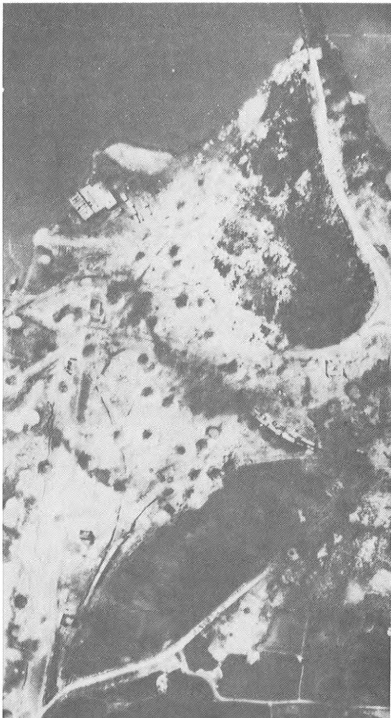
The approach to the Thanh Hoa Bridge (Valley of the Moon).
