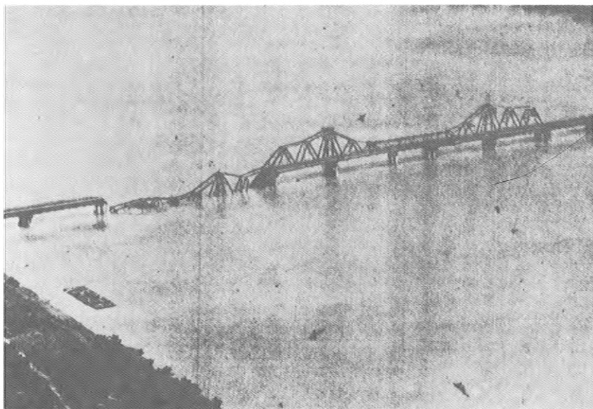
Post-strike photo showing the destroyed spans of the Doumer Bridge after the 10 Sep 1972 strike by F-4s from the 8th Tactical Fighter Wing.
