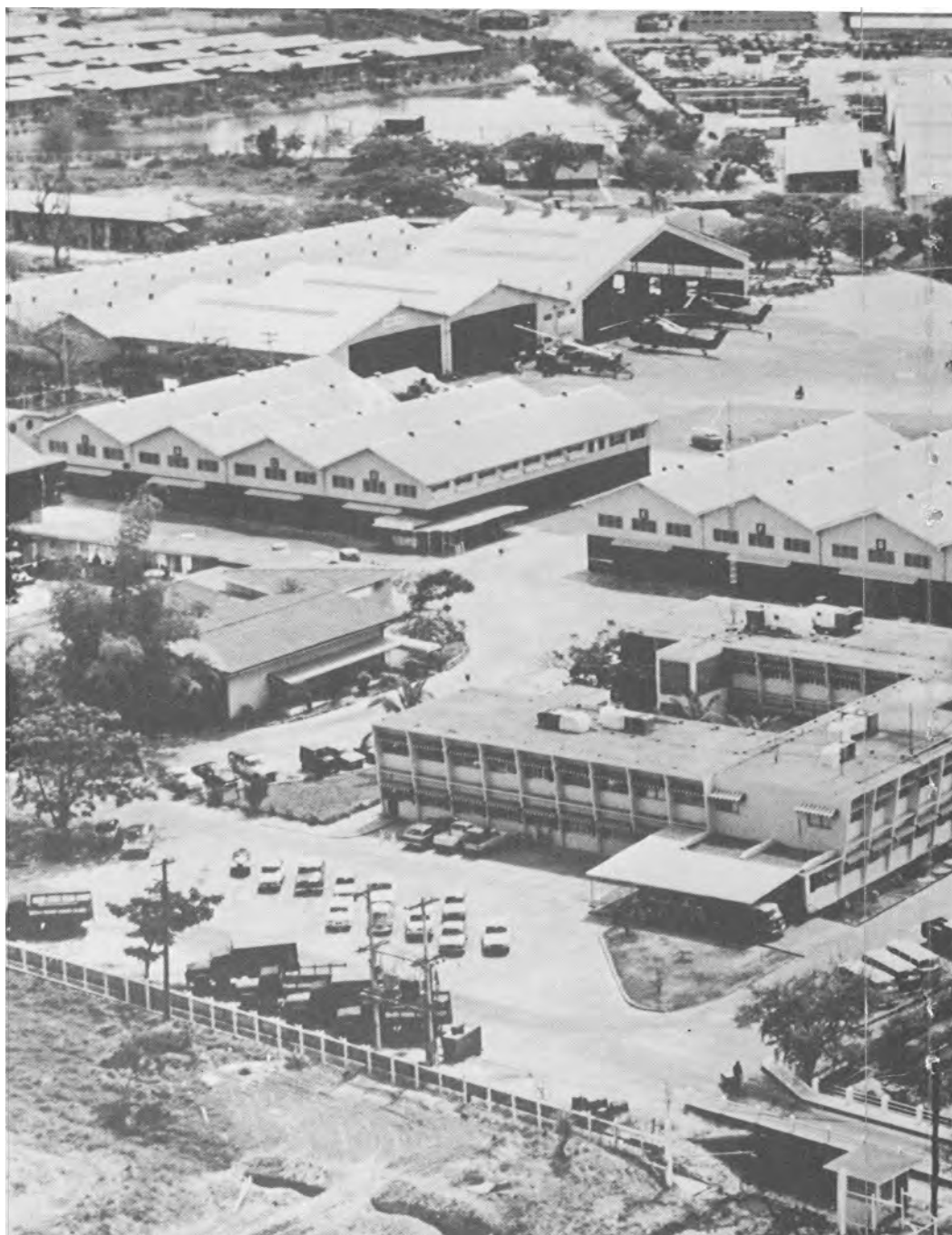
Air America headquarters, Udorn Air Base, Thailand.
