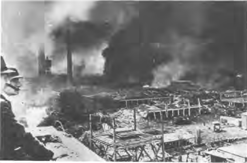
A captured German photo of damage to the Fieseler aircraft plant, Kassel, Germany, after RAF and Eighth Air Force raids.
