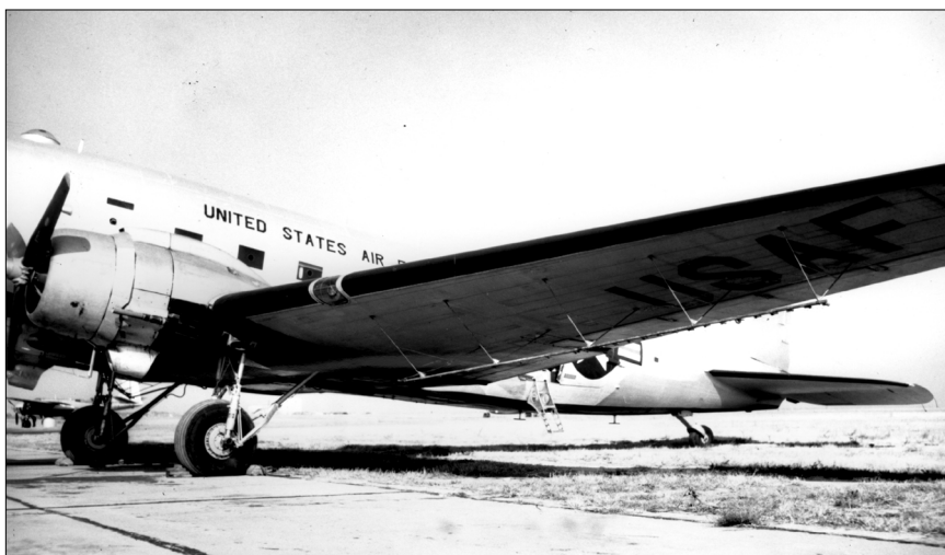
A Douglas C-47 is modified with special boom-type spray equipment attached under the wings to more effectively apply insecticide over areas threatened by the devastation of Hurricane Diane in 1955. (NARA photo.)
