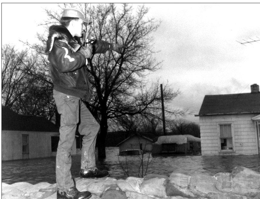
An airman uses a walkie-talkie to direct work on the construction of a sandbag dike to control rising floodwaters near Grand Forks AFB, North Dakota. (NARA photo.)
