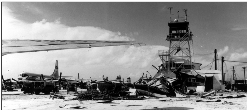
Airfield damage on Wake Island was severe in the aftermath of Typhoon Olive. The island rises only 15 feet above sea level. (NASM photo.)
