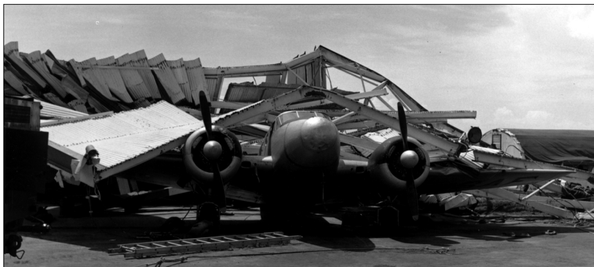
An Air Force C-45 suffered major damage when a roof collapsed on it at Central AB, Iwo Jima, during the onslaught of Typhoon Louise in September 1955. (NARA photo.)
