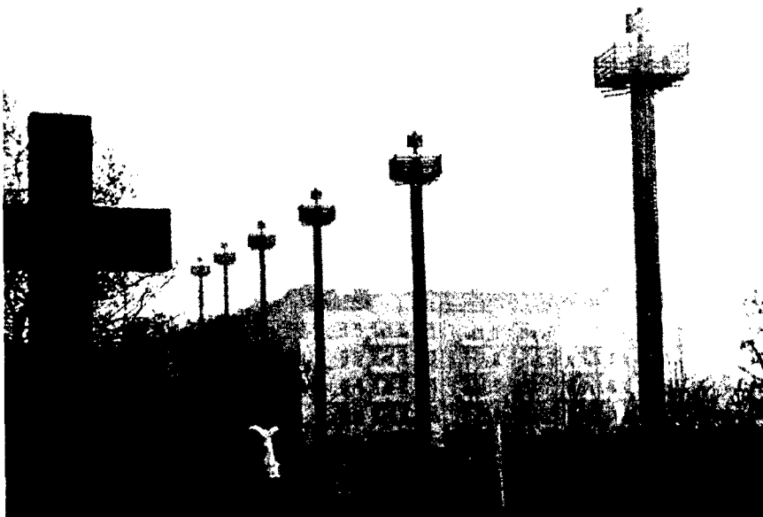
“Airfield lighting arrangements at Tempelhof.” A 200,000-watt system of high intensity approach lights placed in a cemetery illuminated a 3,000 foot approach to the main runway at Tempelhof. ( U.S. Air Force. )
