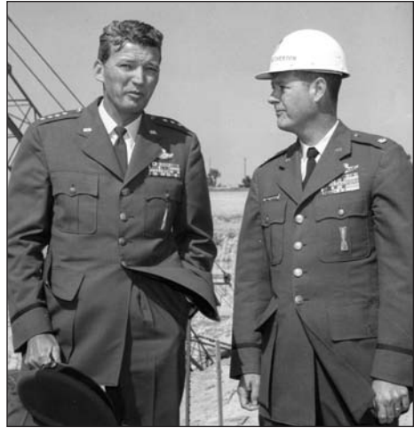
A hands-on manager, General Schriever inspects the construction site at Vandenberg AFB, accompanied by Col. Nether-ton.
