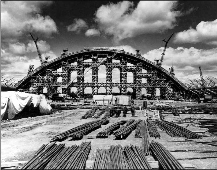
A B-36 hangar under construction in 1948 at Limestone (later, Loring) Air Force Base, Maine, the first new Strategic Air Command base.
