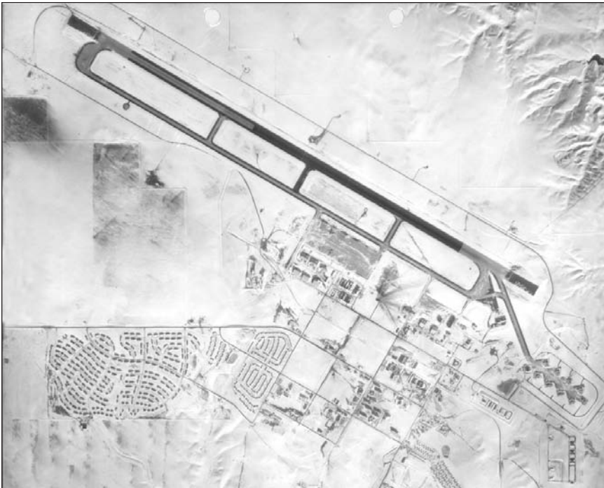
Aerial view of Glasgow Air Force Base, Montana, originally constructed from scratch as an ADC base in the northern tier states during the 1950s, which eventually served as a major SAC base in the 1960s.
