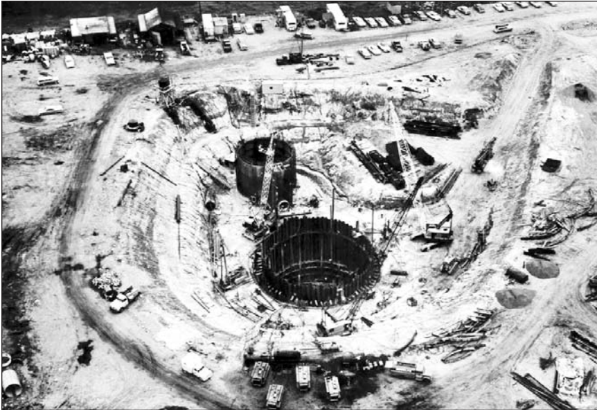
Construction site, early 1960s, for the Series F Atlas ICBM “silo-lift” launcher at Plattsburgh Air Force Base, New York. On a “silo-lift” launcher, the missile is stored vertically within a hardened, underground silo.
