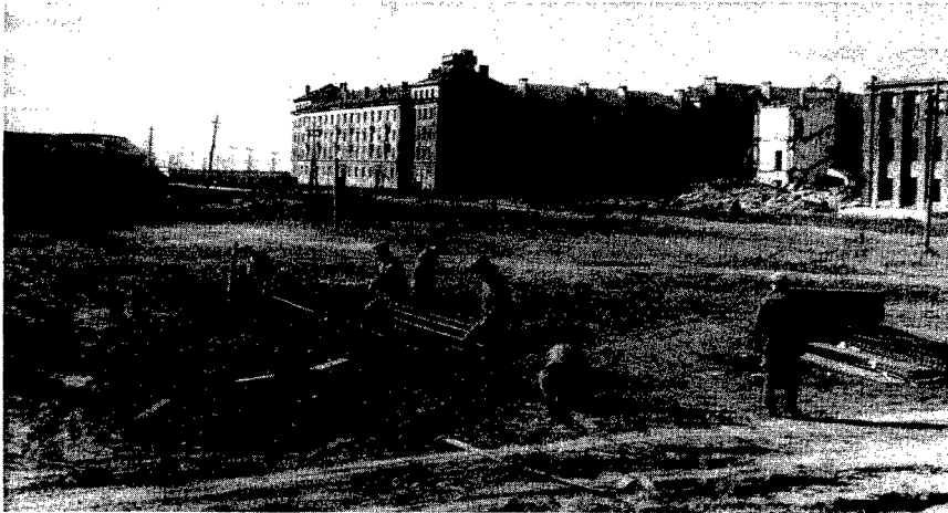
American aviation engineers lay out pierced steel plank runways at Poltava in the spring of 1944.
