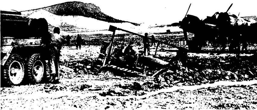
D-7 bulldozer fills crater torn into a North African airfield. Rapid repairs ensured near continuous operations.
