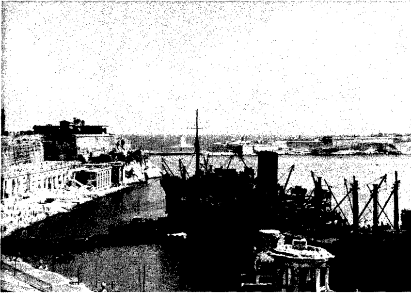
Grand Harbor, Malta. Damage to dockside structure at left is evident; bomb throws up spray beyond the harbor breakwater. Imperial War Museum
