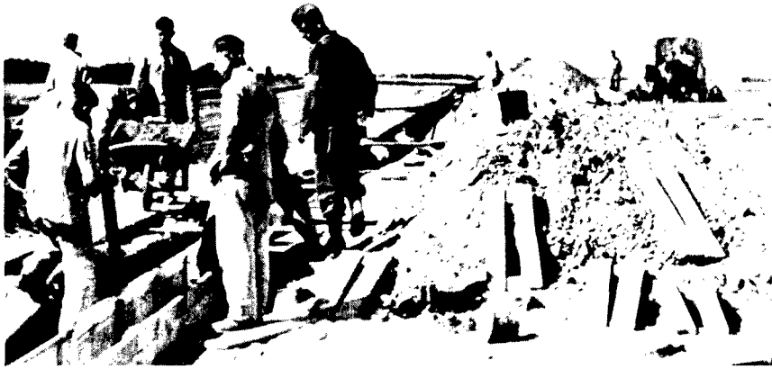
German airfield construction in Russia, 1941. Reich Labor Service battalions pour footings and emplace primitive but durable wood stump taxiways.
