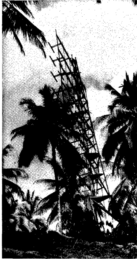
The SCR-270 radar had ten degrees of tilt designed into its frame. Master Tech. Sgt. Dermott H. McDonnell used this feature to advantage in the defense of Guadalcanal.
